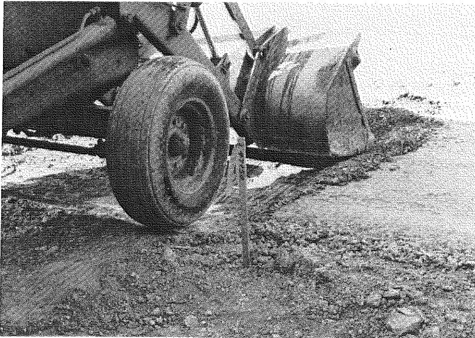
Figure 10. Cutting gaps in the first lift of the AFBC concrete base.
