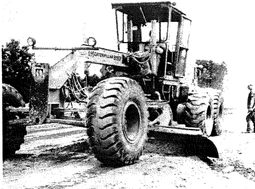
Figure 19. A road grader was used to trim the modified subgrade to elevation grade.
