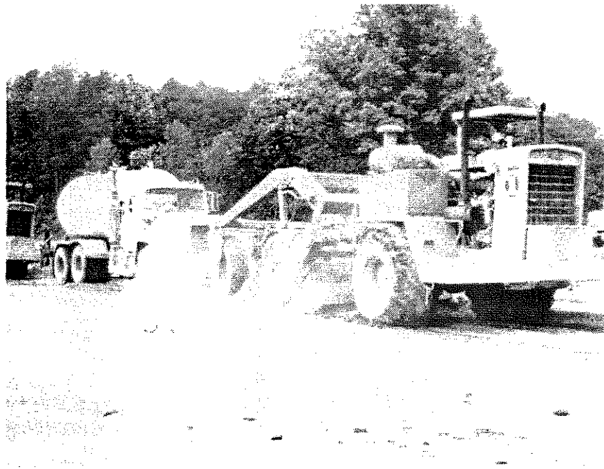
Figure 17. A soil pulverizer mixes the AFBC spent lime with the natural soil. A water truck adds water necessary to achieve proper moisture content.
