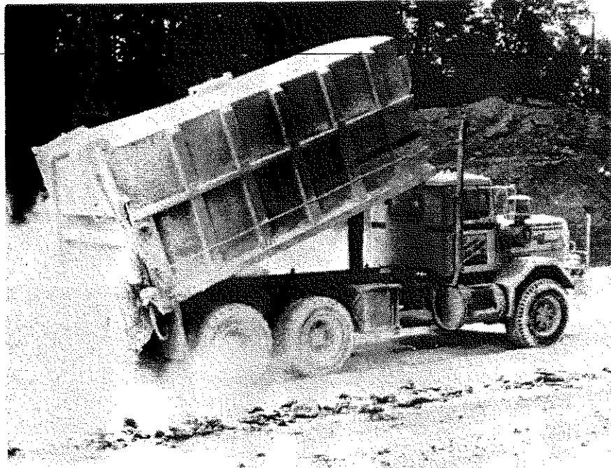
Figure 16. Spreader truck distributing AFBC spent lime materials over the surface of the prepared subgrade.
