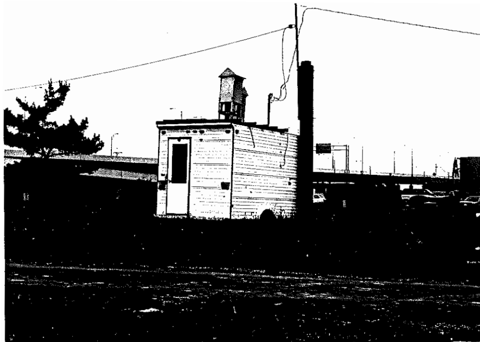
Figure 2. Total Suspended Particulate Monitor Mounted atop a Portable Shelter.
