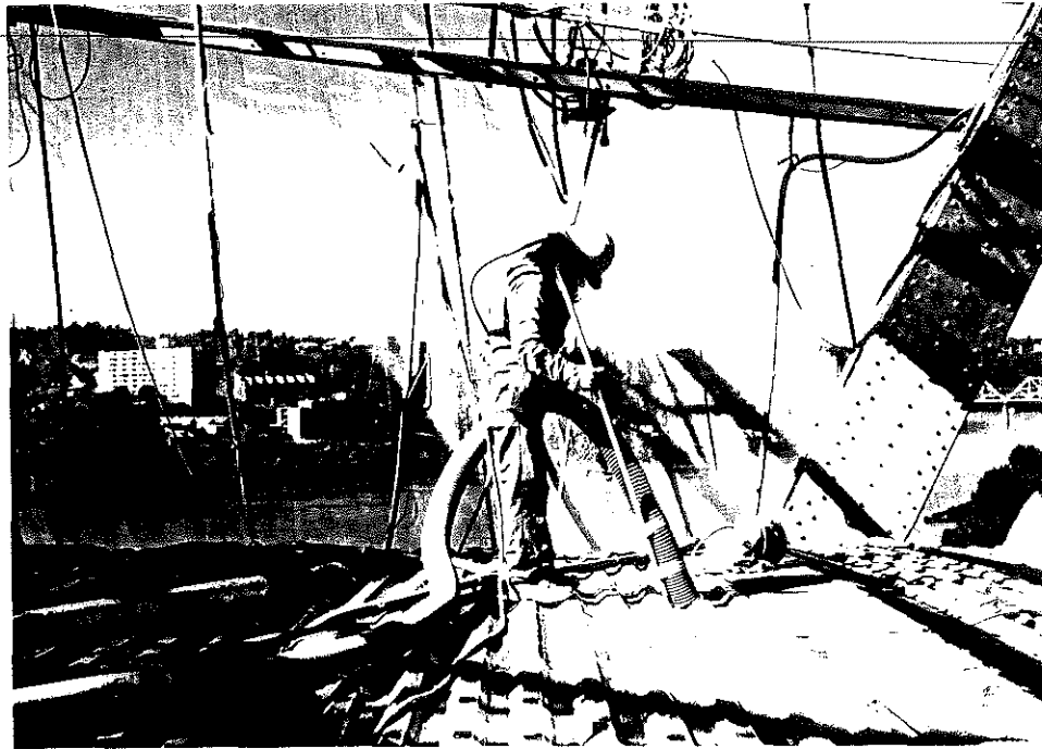
Figure 3. Worker inside a Containment Enclosure Wearing an Air-Supplied Helment.
