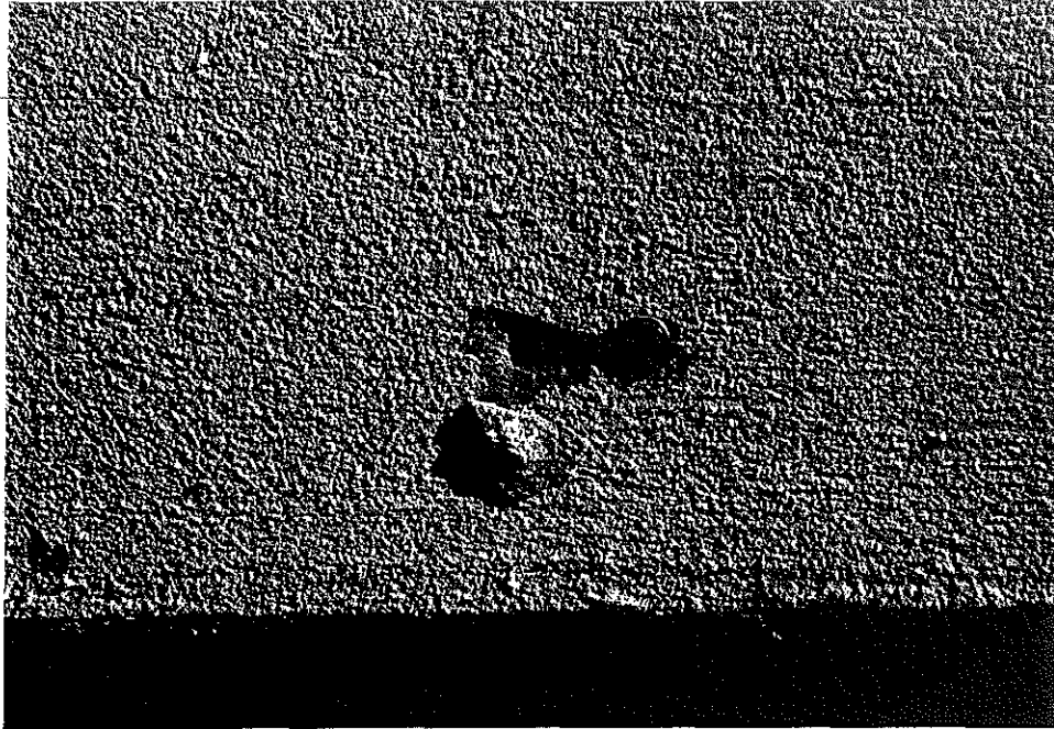
Figure 6. A fractured aggregate particle dislodged from the Class S concrete barrier wall.
