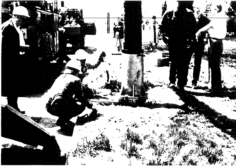
Figure 13 - Add Slip Plate, Bolts, Washers, Nuts, and Torque to 200 Ft-Lb
