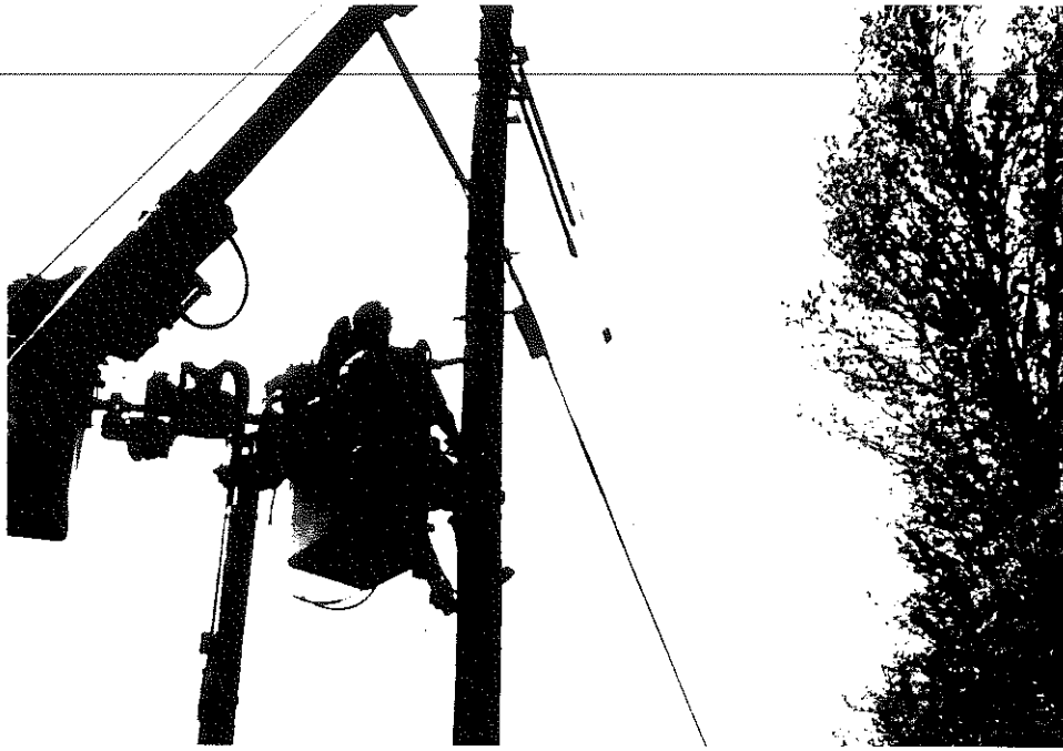
Figure 15 - Drill through Pole
