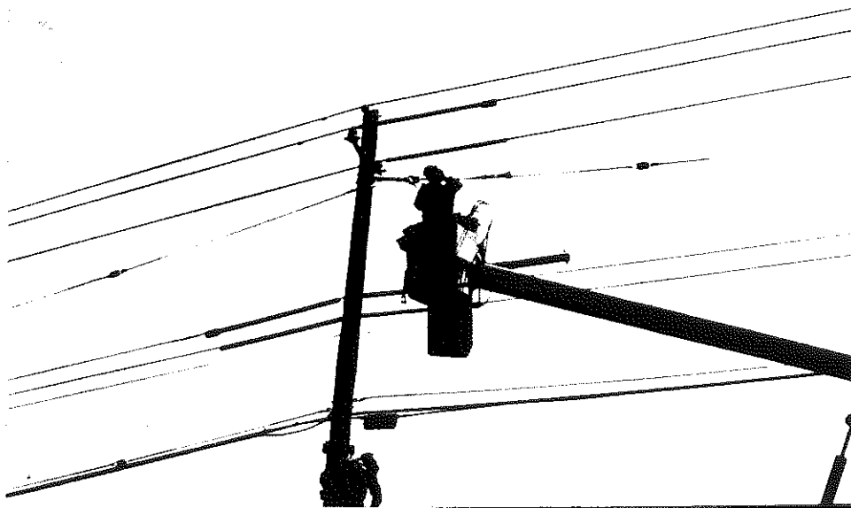
Figure 6 - Insulate Lines
