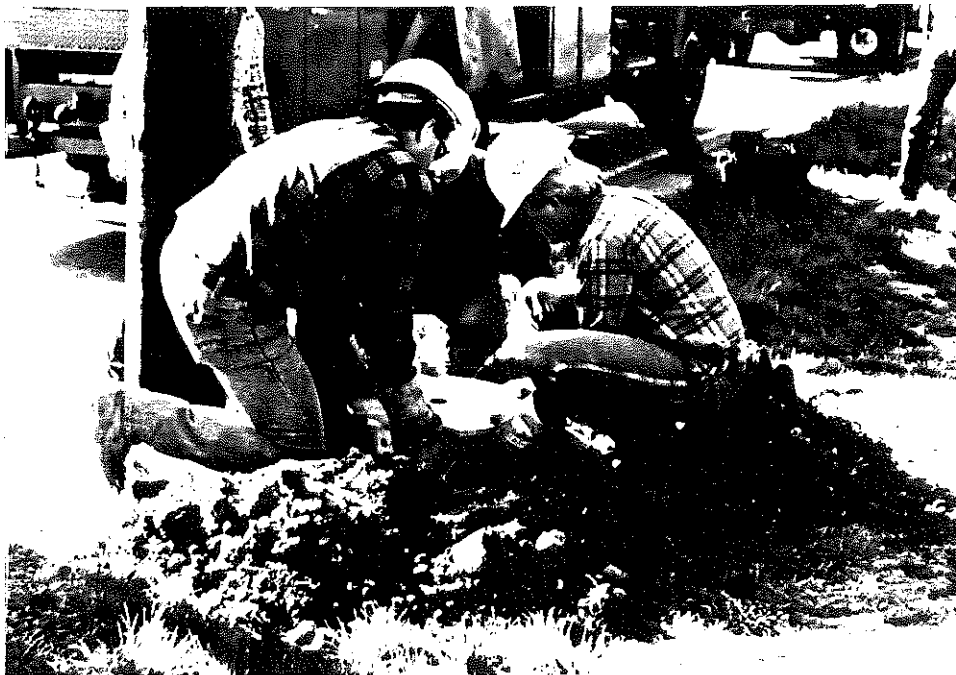
Figure 10 - Install Lower Tube with Base
