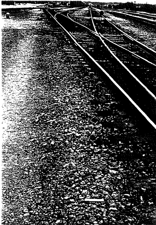
North End of C Yard, Ladder Track
