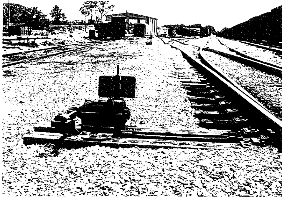
South End of Yard, Looking Compass East
