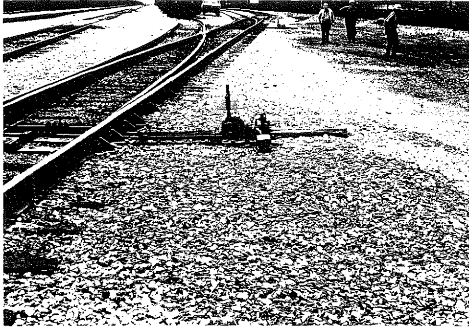
West Yard, North End No. 3 Track at Lead
