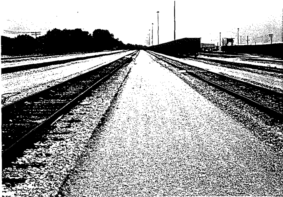
West Yard, Between No. 4 and No. 5 Tracks Paved Walk/Driveways
