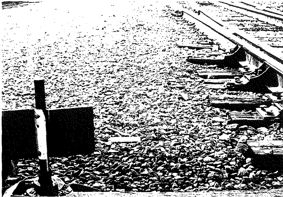
No. 2 Lead, West End of East Bound Yard
