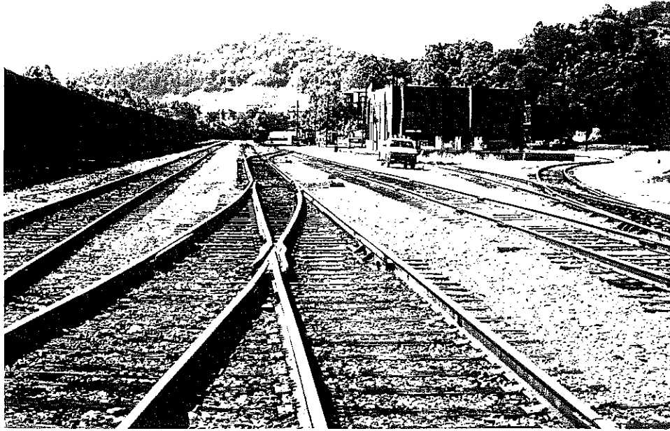
Overview of Hazard Yard
