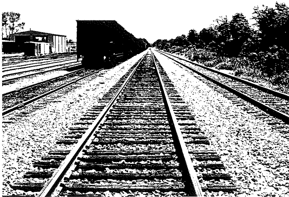
Mainline Adjacent to Yard
