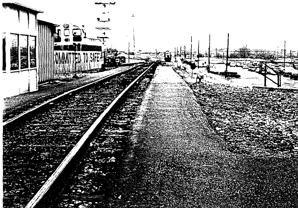
Paved Hump Track
