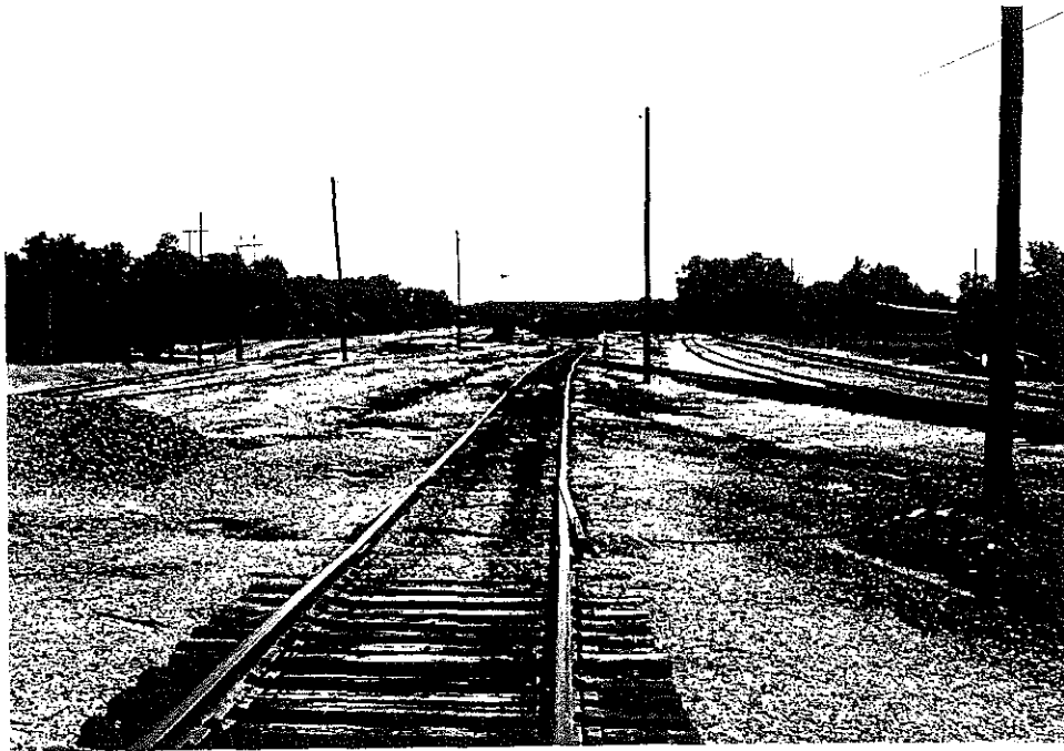
South Yard, Looking South
