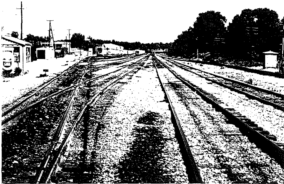
North Yard at South End Looking North
