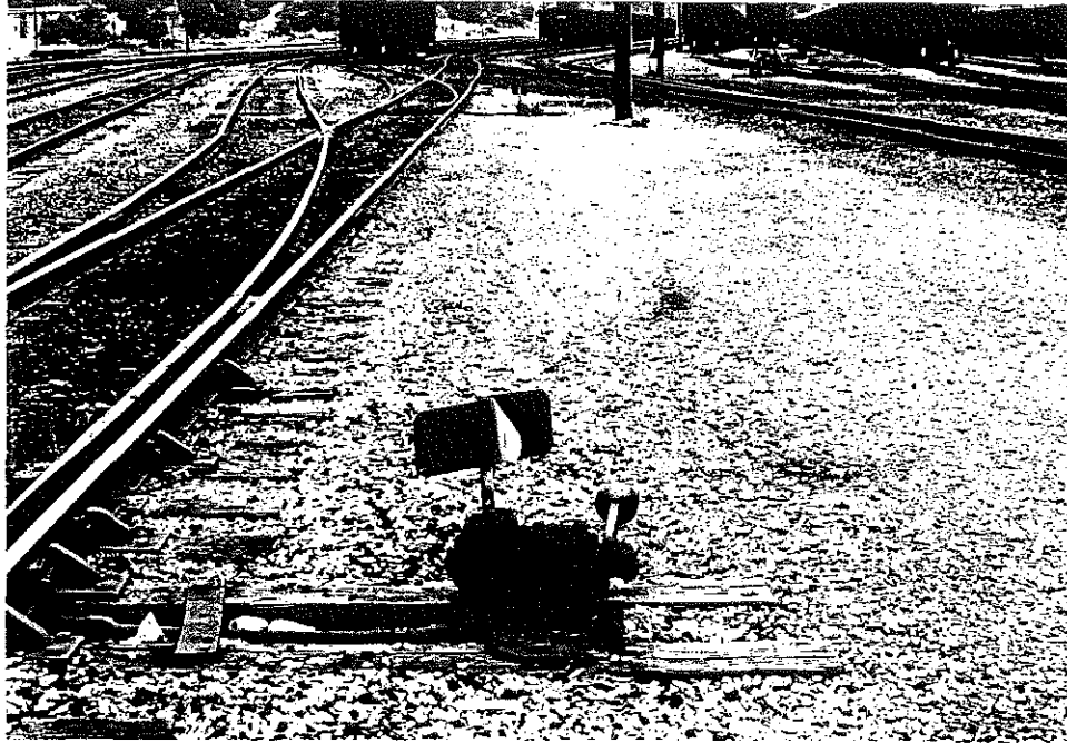
South End of Yard Looking North
