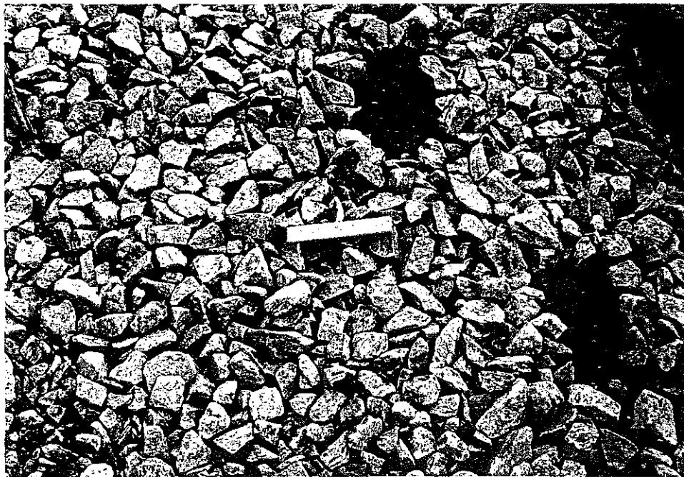
Close Up of North End of Mapother Yard, Large Ballast
