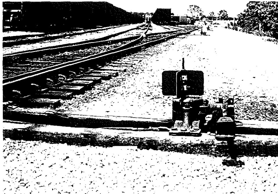
Ladder Track at North End of Yard, Looking Compass West
