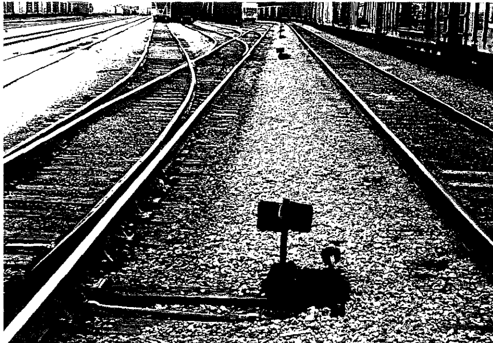
South End, No. 8 Track at Ladder Track
