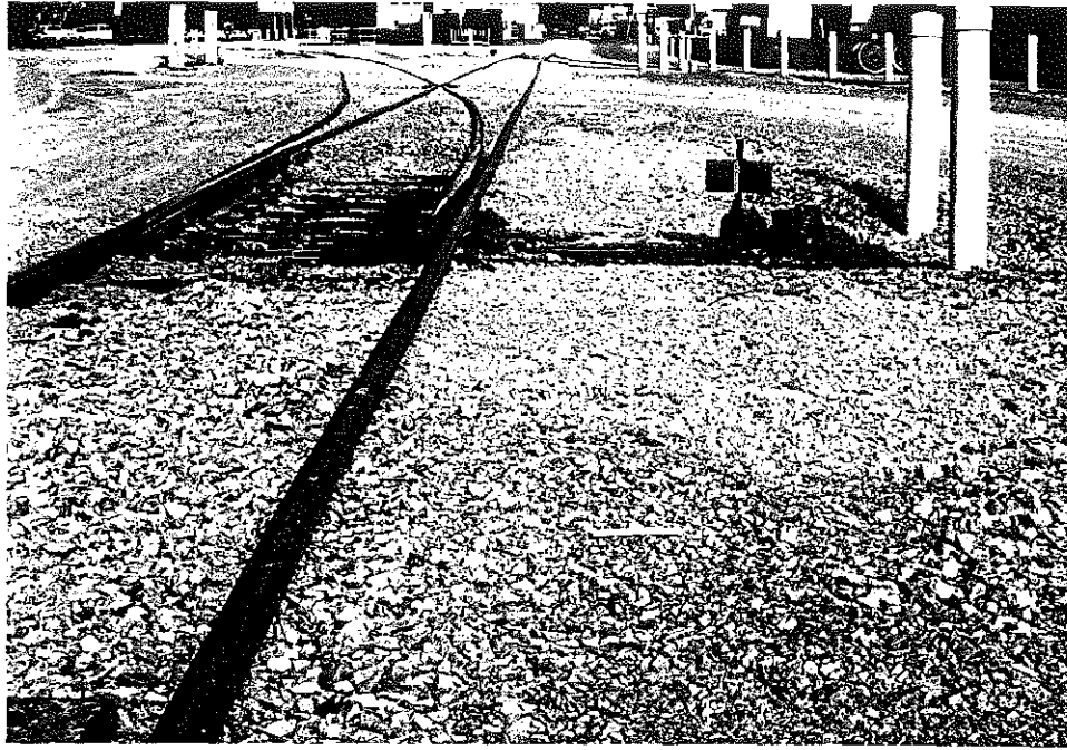
Car Shop, Throughfare Track
