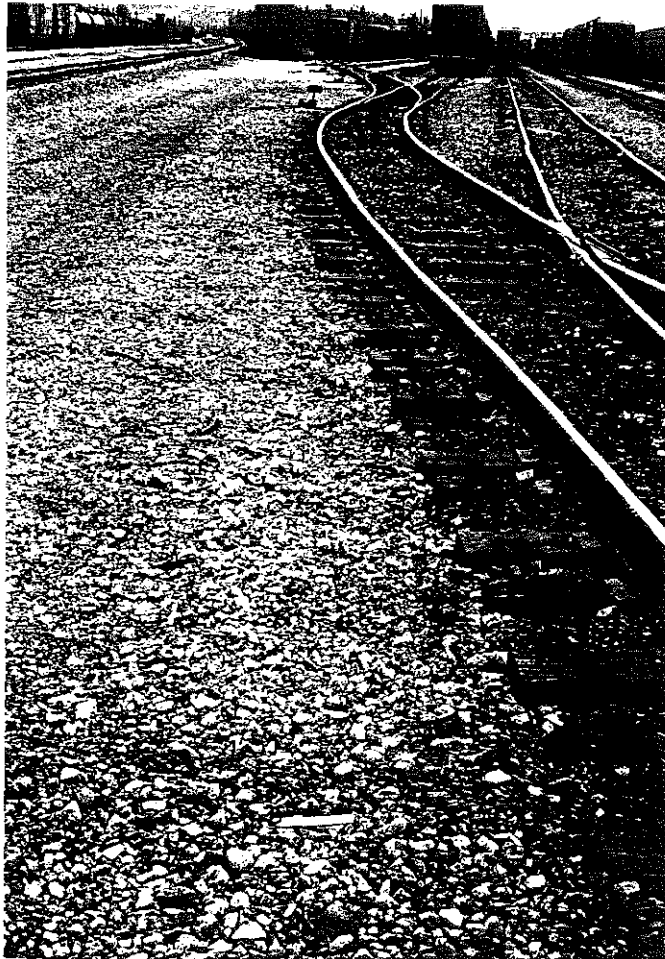
Ladder Track North End of N Yard
