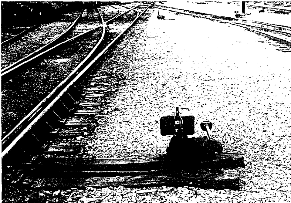
North End, No. 11 Track at Ladder Track
