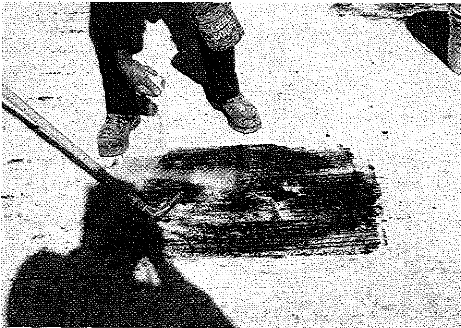
Figure 6. An epoxy compound was spread on the ground spots and sand was applied for surface texture.
