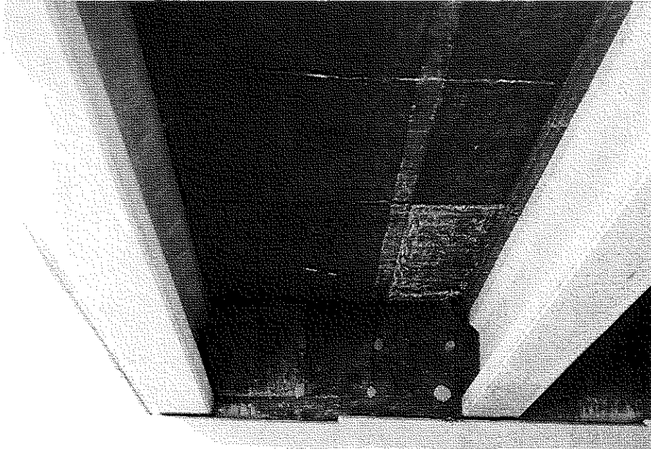
Figure 9. Full-depth cracking of the control deck viewed from beneath the deck.
