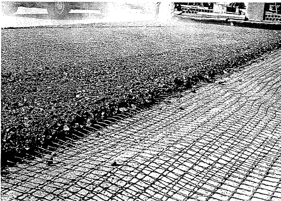
Figure 7. Waves developed between the paver and the haul truck.
