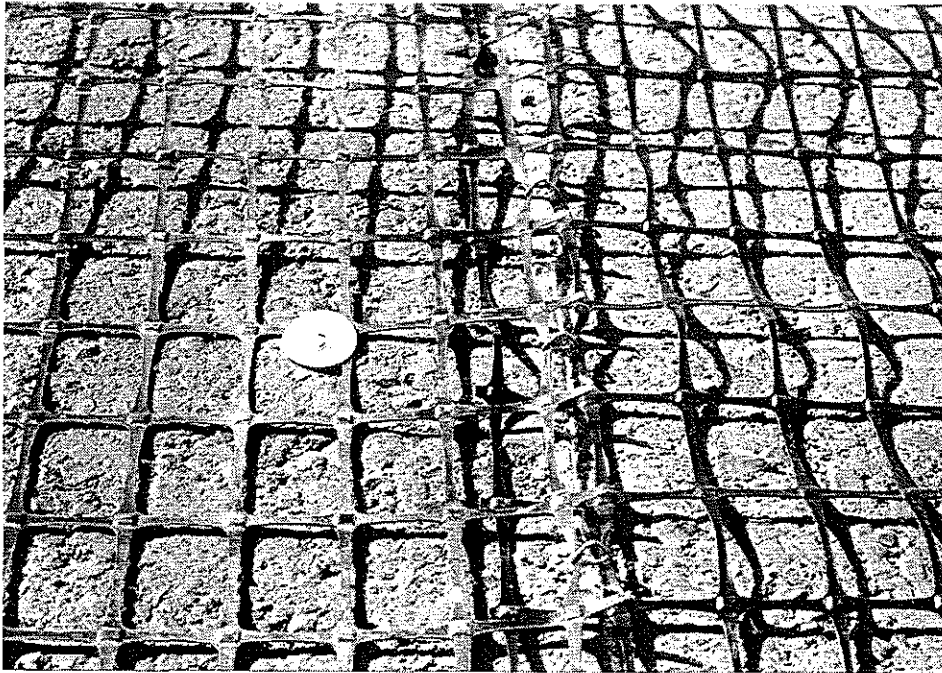
Figure 6. Pinning the reinforcing grid to the base course.
