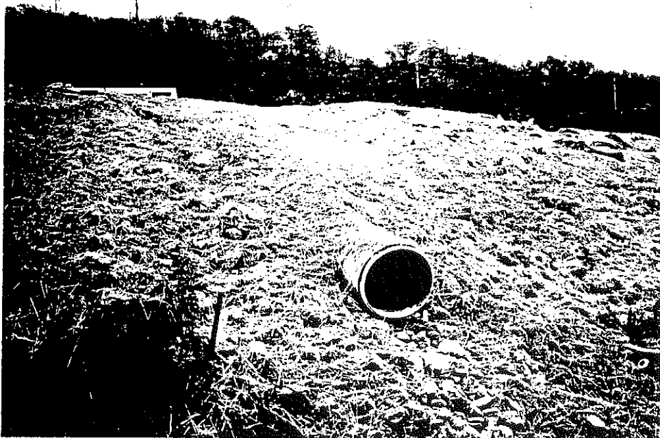
Figure 8. Outlet End of PVC Pipe at Station 129+72
