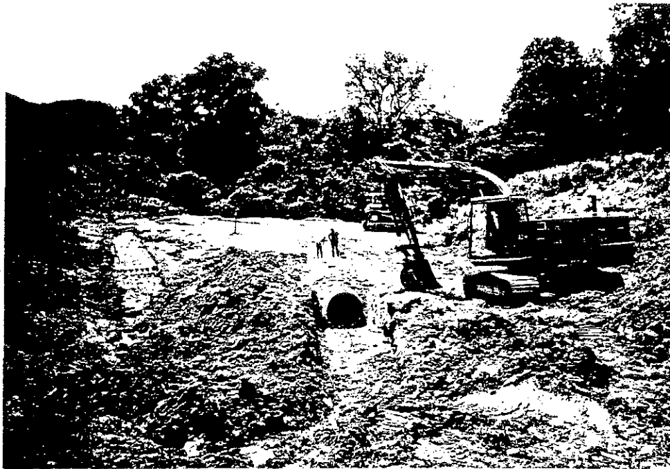
Figure 4. Installation of 1.2m Pipe at Station 104+70
