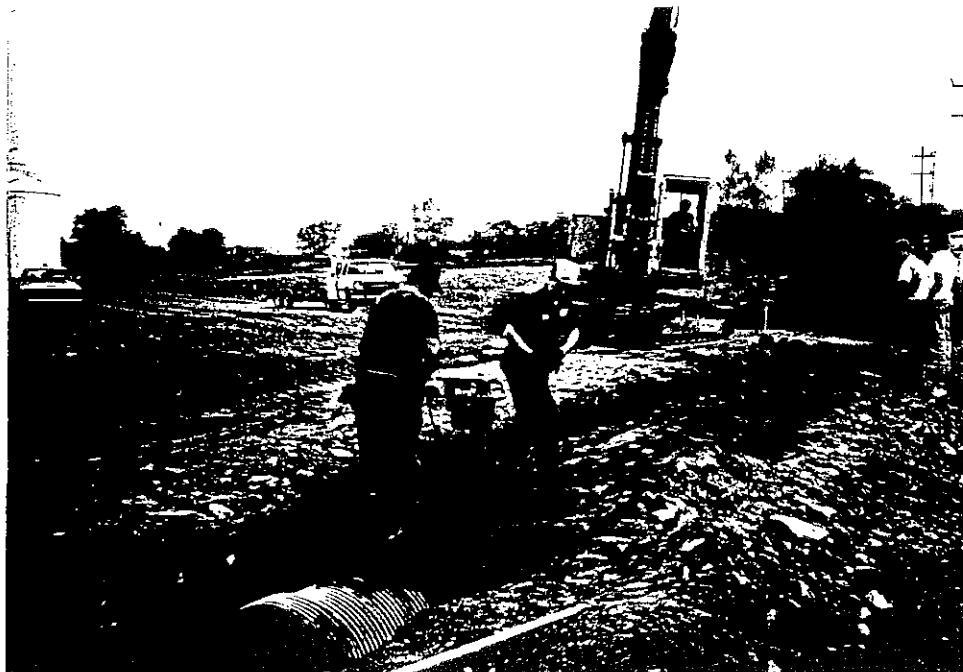
Figure 5. Installation of 0.76 m Pipe at Station 162+00
