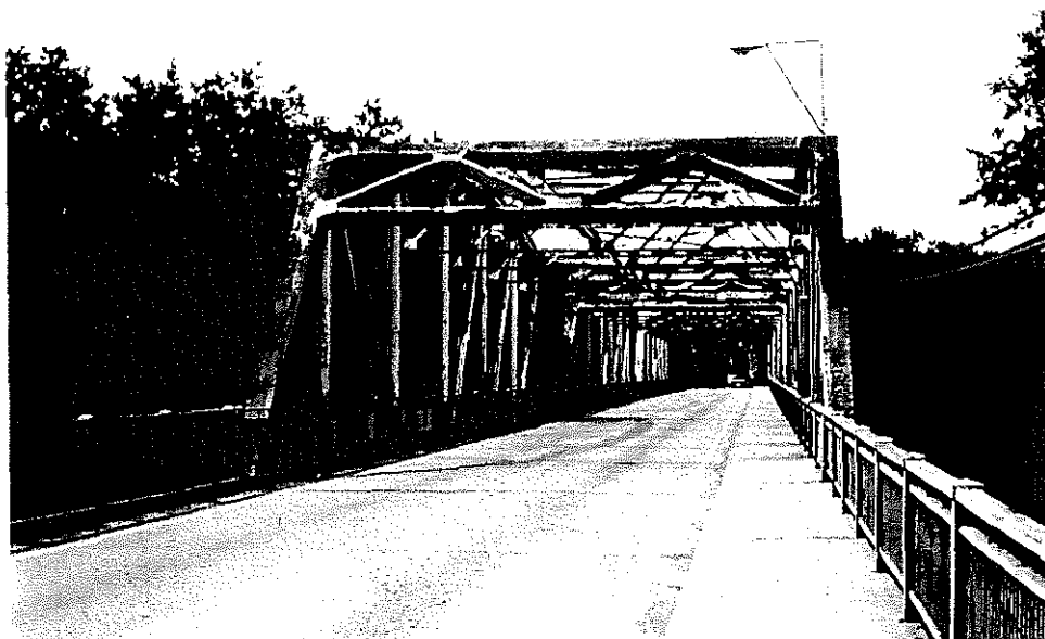
Figure 5. Initial Condition of the KY 177 Bridge Showing Severe Weathering of the Alkyd Topcoat (1992).
