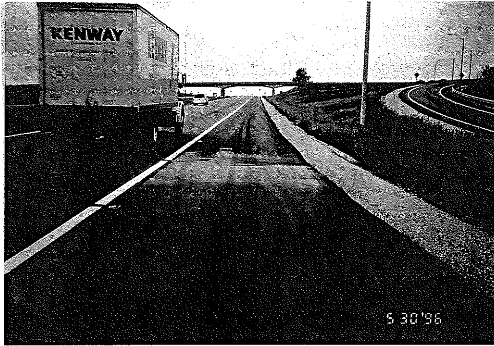
FIGURE 1. SIGNS OF PUMPING AT SHOULDER CONSTRUCTION JOINT.
