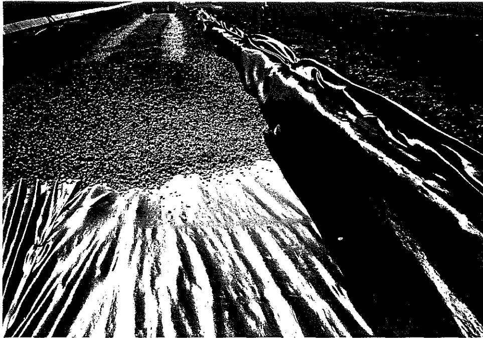
Figure 18a. Bridge end drainage being installed.
