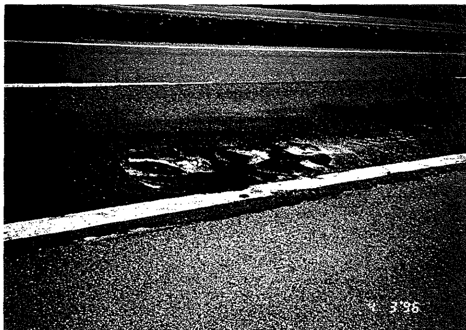
Figure 20a. Signs of water induced failure in asphalt pavement.
