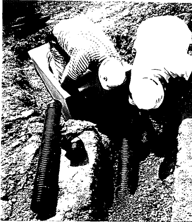
Figure 5a. Construction photo showing single wall flexible pipe coming from headwall being attached to double wall outlet pipe. Research indicates that most of the damage occurs in the flexible pipe “pigtail” coming from the headwall.
