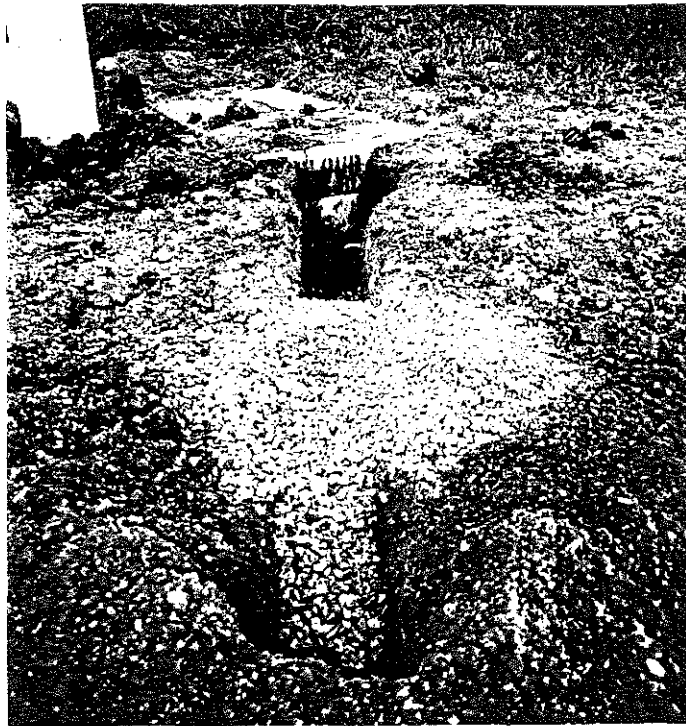
Figure 6. Outlet pipe being backfilled on Interstate 64.
