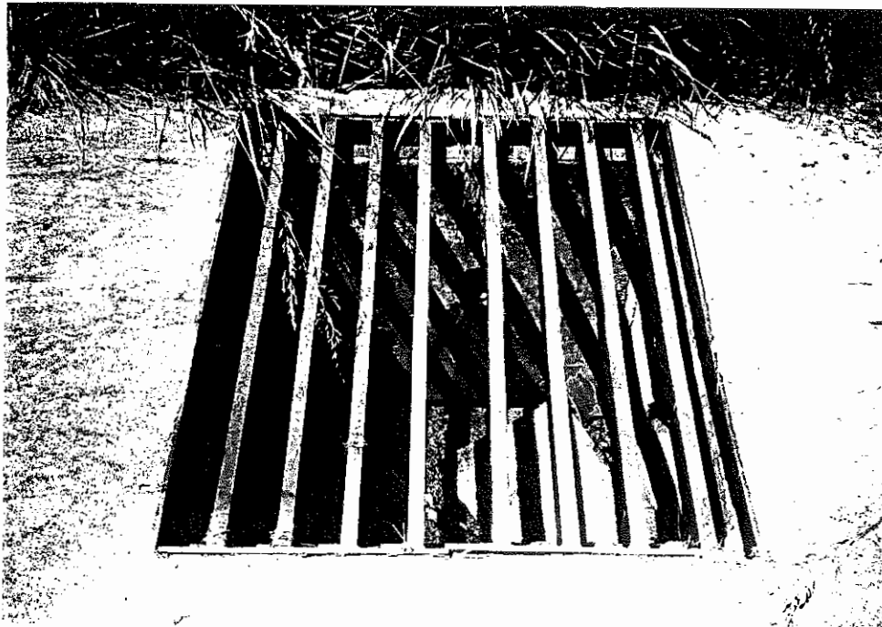
Figure 2. Edge drain outlet cut into drop box (no rodent screen).
