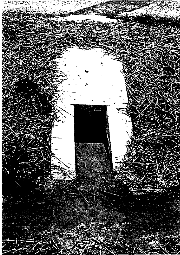
Figure 13a. Headwall installed in shallow ditch line.
