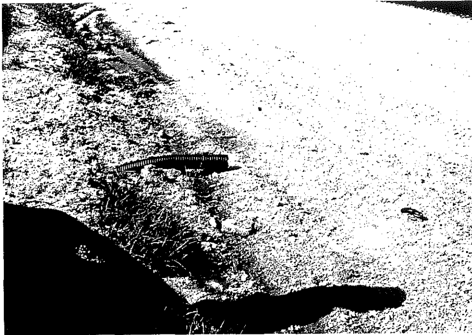
Figure 7a. Outlet pipes damaged during raising of the shoulder.
