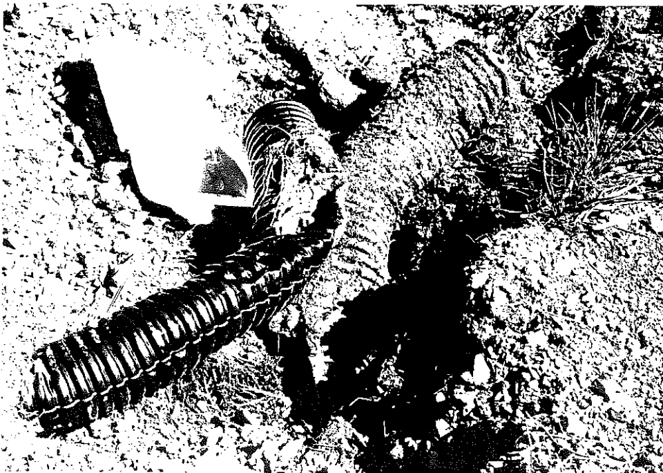
Figure 7b. Outlet pipes crushed prior to headwall placement.
