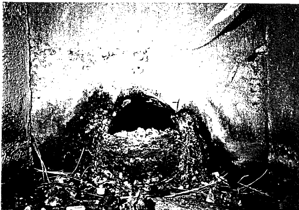
Figure 19c. Partially clogged outlet pipe.
