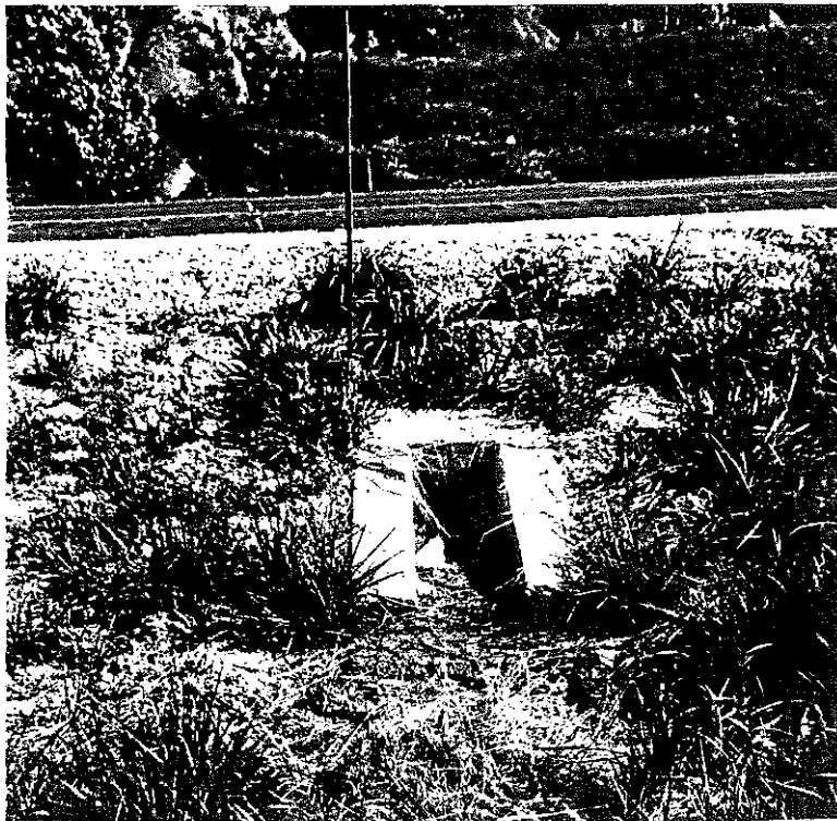
Figure 22. Outlet location marked with delineator post.
