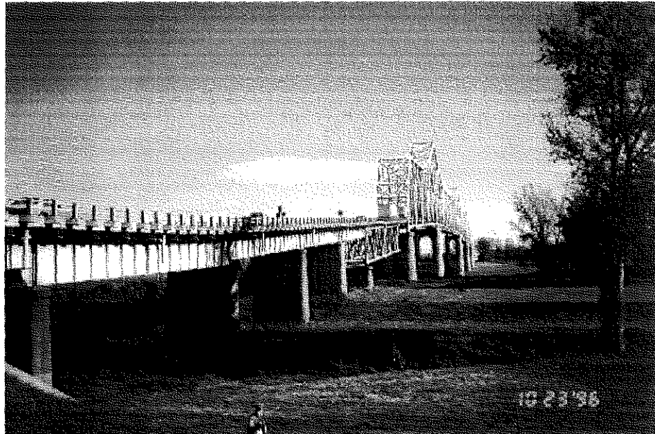
2.1c Illinois approach and end view of the main bridge
