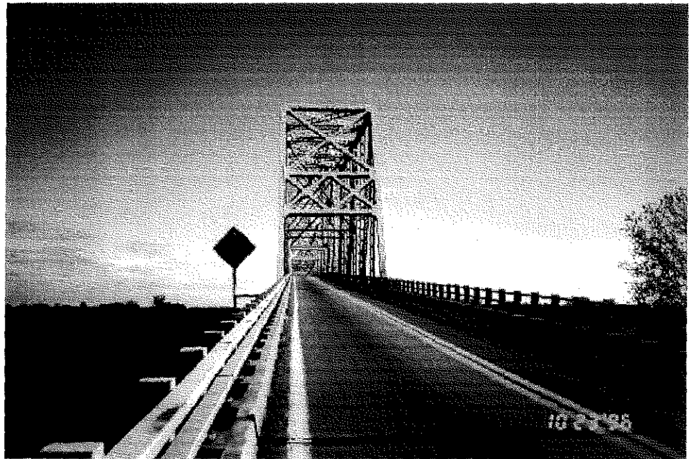
2.1d End portal of the main bridge
