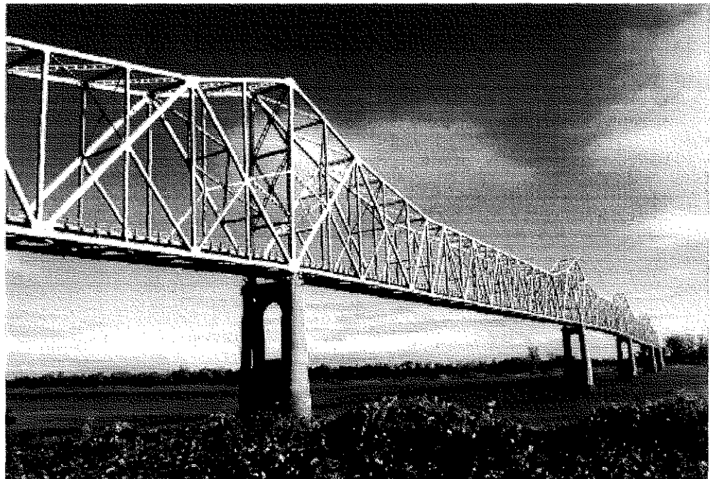
2.1b US51 main bridge across the Ohio river
