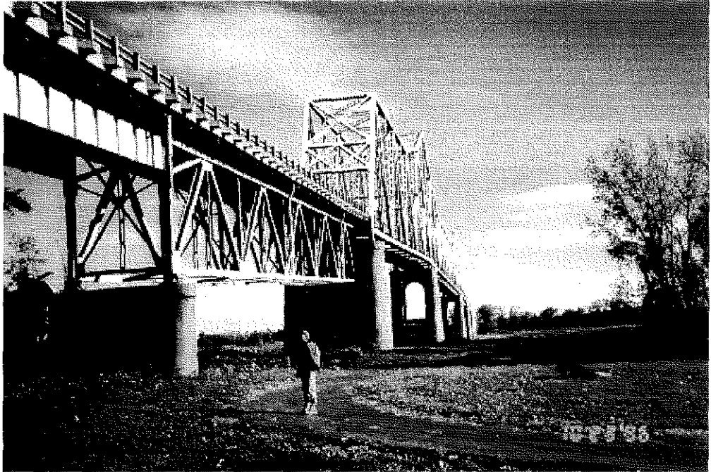
2.1a View showing Illinois approach and US51 main bridge
