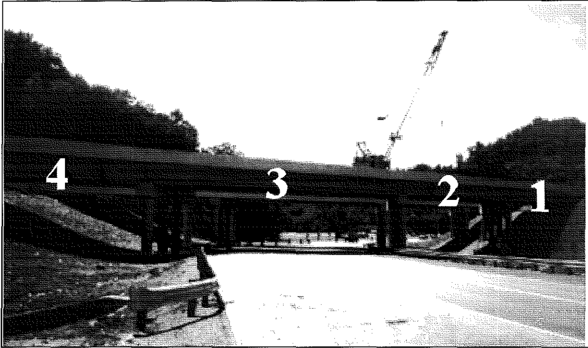
Figure 2.2. US 23 Bridge Over KY 40 (Span Numbers Are Marked - Northbound Traffic Travels from Right to Left [←]).
