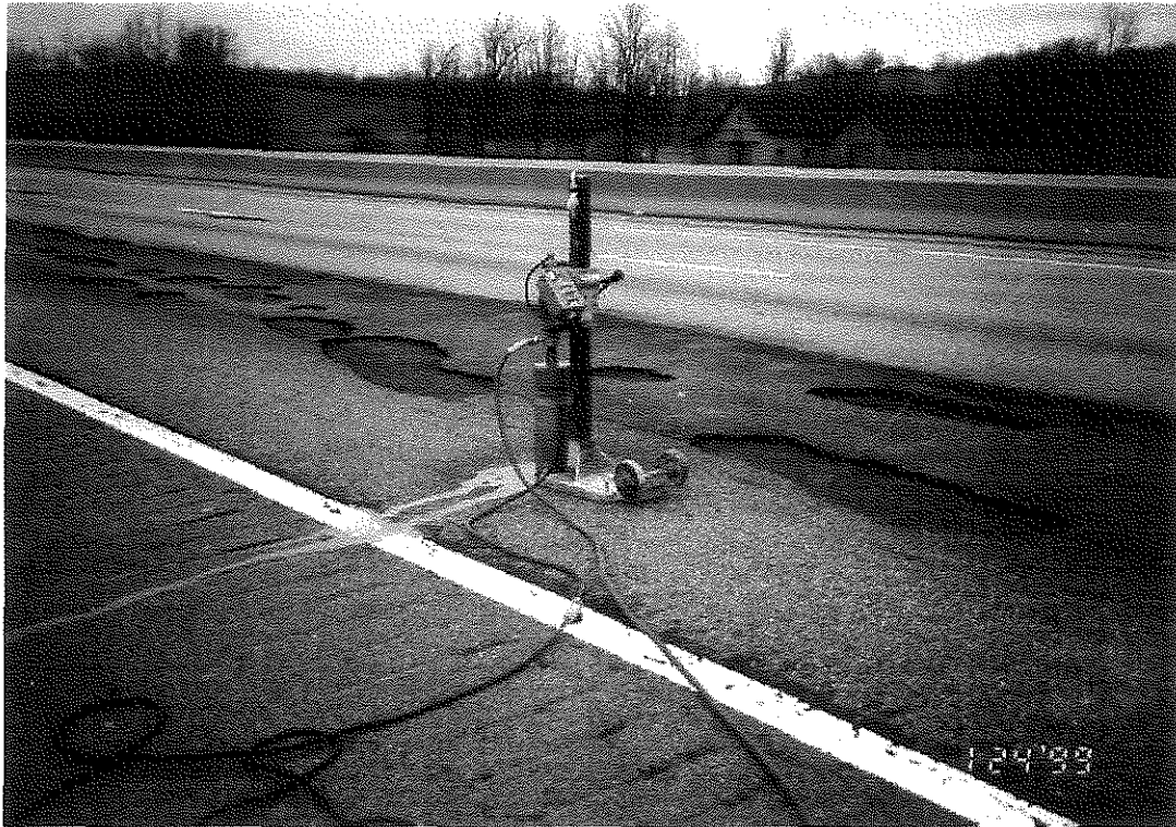
Figure 3. Cores Being Taken in Outside Lane in Delaminated Area.
