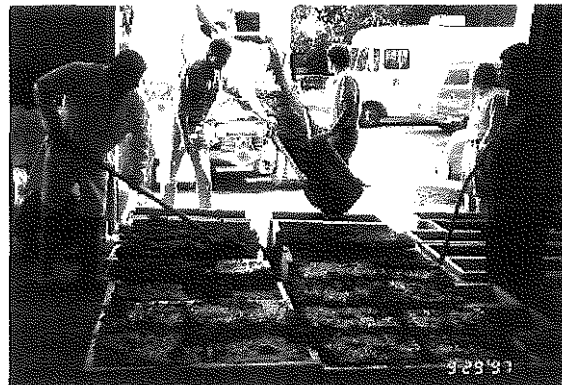
Figure A.5 Concrete Blocks Casting
