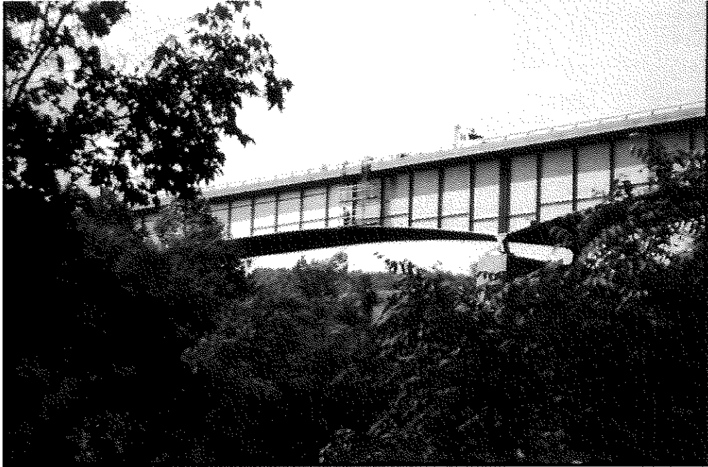
FIGURE 15. TWO-LEVEL SCAFFOLD USED IN PAINTING MAIN GIRDERS ON THE I-64 BRIDGES OVER THE KENTUCKY RIVER.
