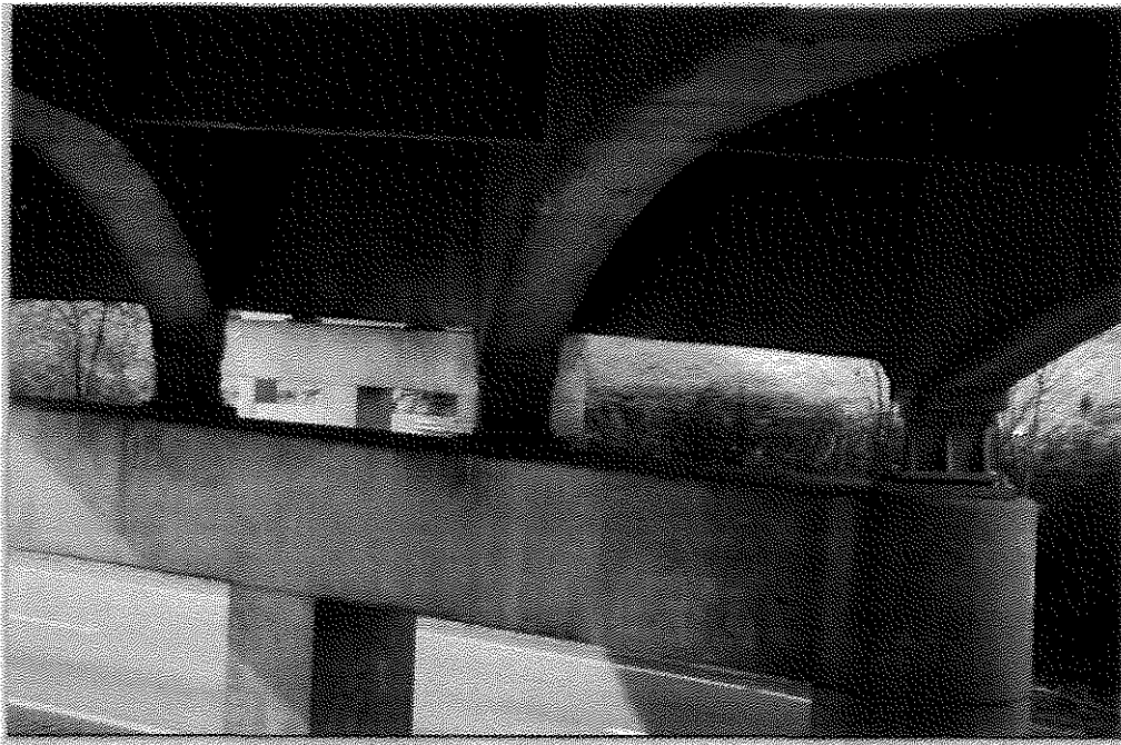
FIGURE 48. I-71 CONCRETE BRIDGE SHOWING PIER BEARING IN GOOD CONDITION (1999).
