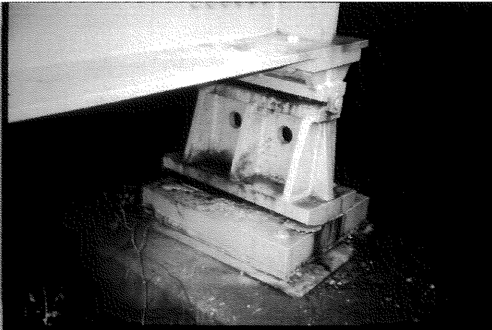
FIGURE 29. I-64 EASTBOUND OVER KY 420 SHOWING BEARING CORROSION (1997).
