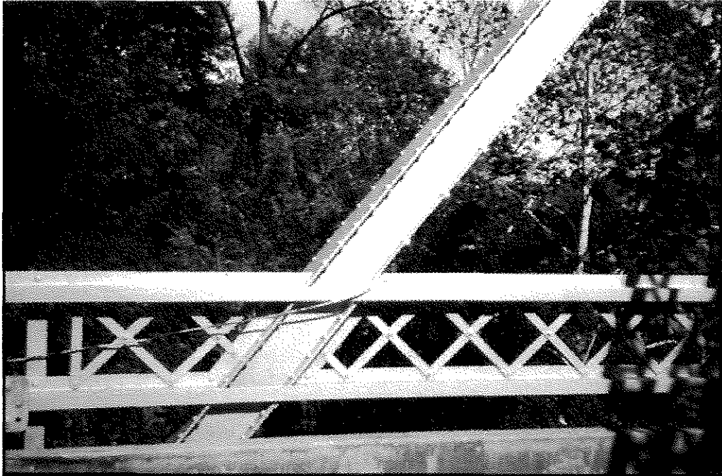
FIGURE 11. FULL PRIME ON END BENT OF THE KY-22 BRIDGE.
