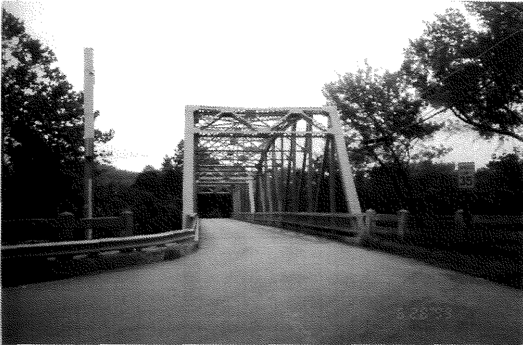
FIGURE 49. NORTH END OF THE KY 22 BRIDGE.
