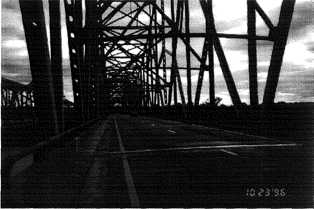
Figure 2.1e Inside View Showing Portals, Cross Bracings, etc
