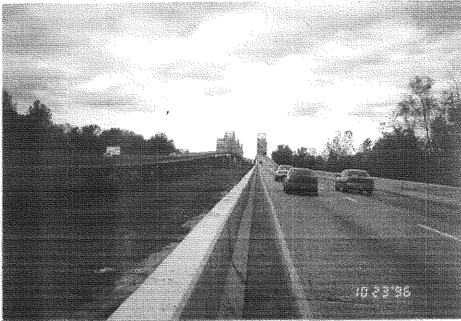
Figure E-2 The US41 Southbound Approach Spans at Henderson, KY
