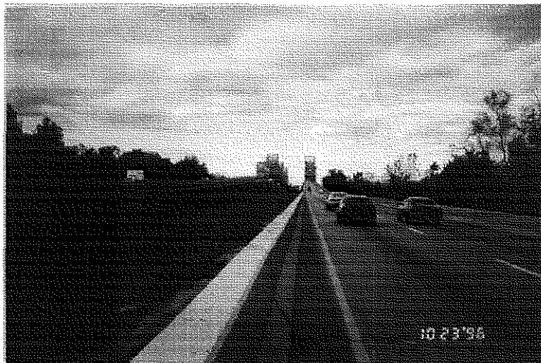
Figure 6.1b Henderson, KY Approach Bridge
