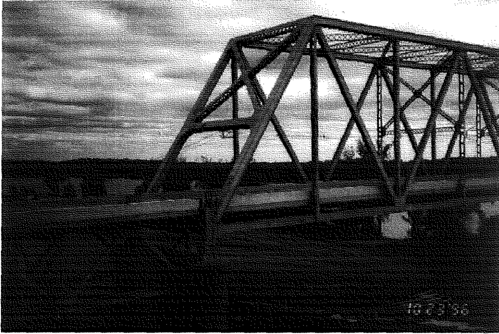
Figure 2.1c End portal of the US41 Bridges
