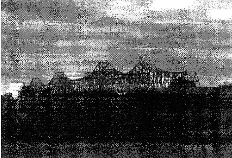
Figure E-1 US41 Bridges over the Ohio River at Henderson, KY
