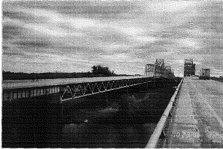
Figure 6.1c View of Evansville, IN Approach Bridge
