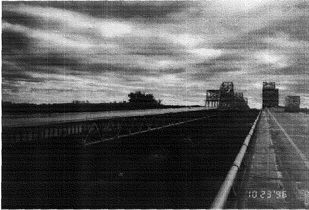
Figure 2.1a US41 Bridges over the Ohio River at Henderson, KY - Entrance View
