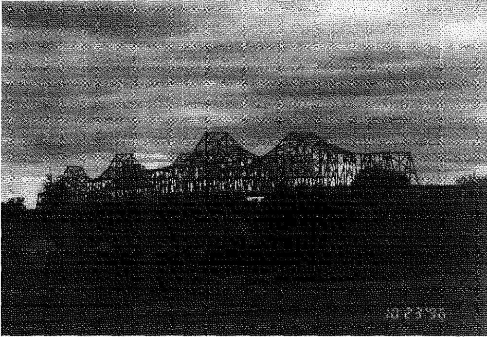
Figure E.1 US41 Bridges over the Ohio River at Henderson, KY
