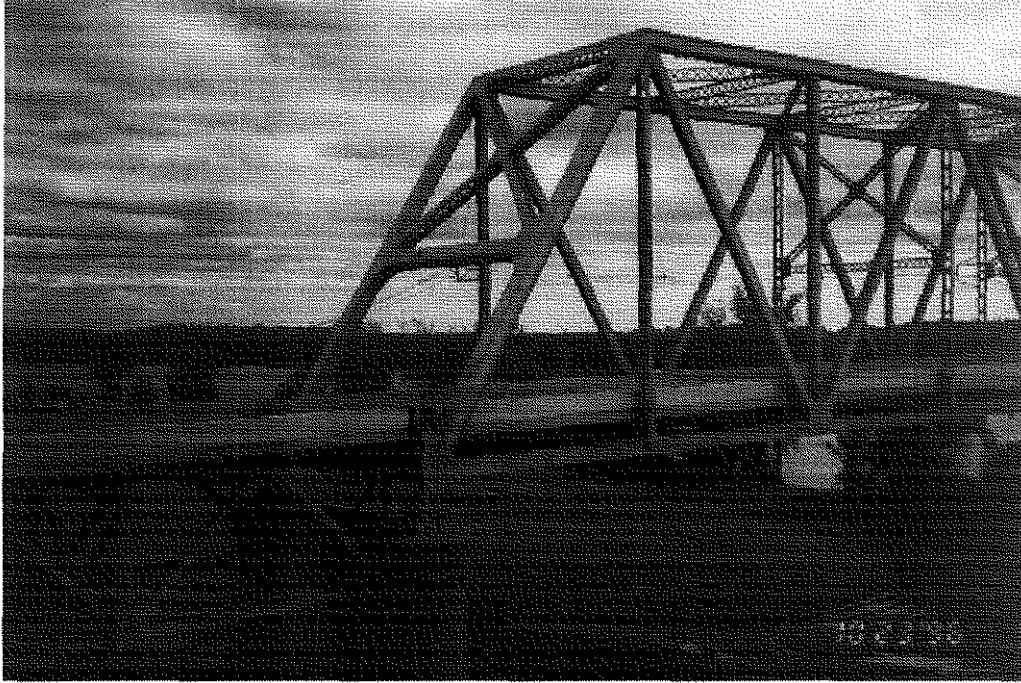
Figure 2.1c End portal of the US41 Bridges
