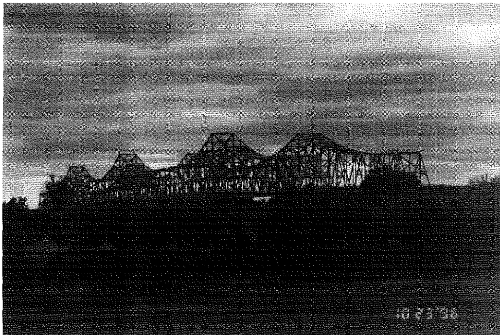
Figure 2.1b Side Views of the US41 Bridges over the Ohio river
