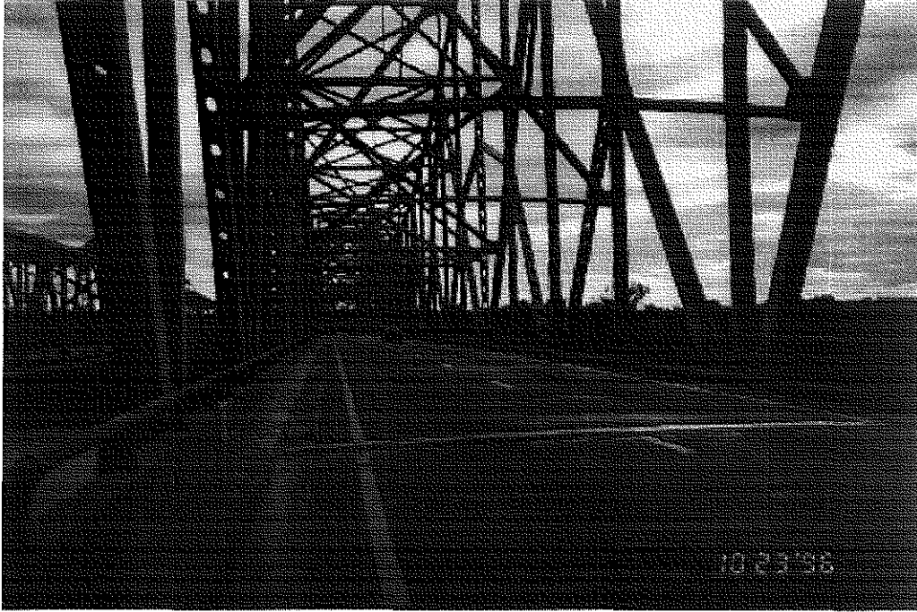
Figure 2.1e Inside View Showing Portals, Cross Bracings, etc
