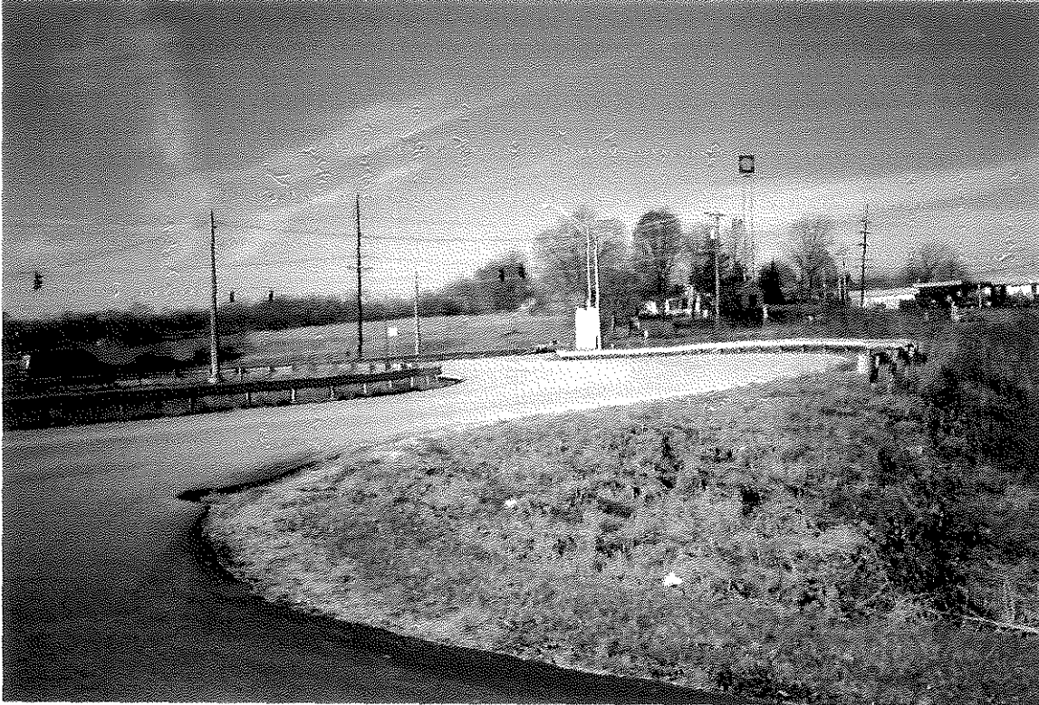
Figure 5: Westbound View of Curvature on Chenault Road (near US 60)
