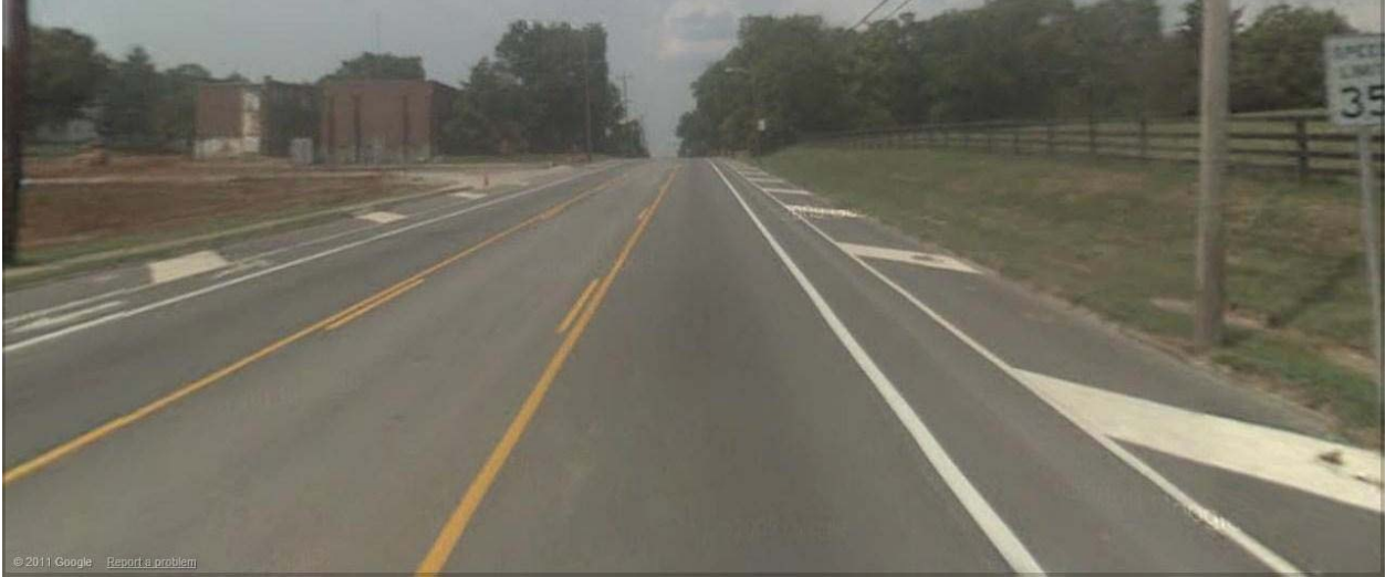
Figure 5: US 60 with Added Shoulders
