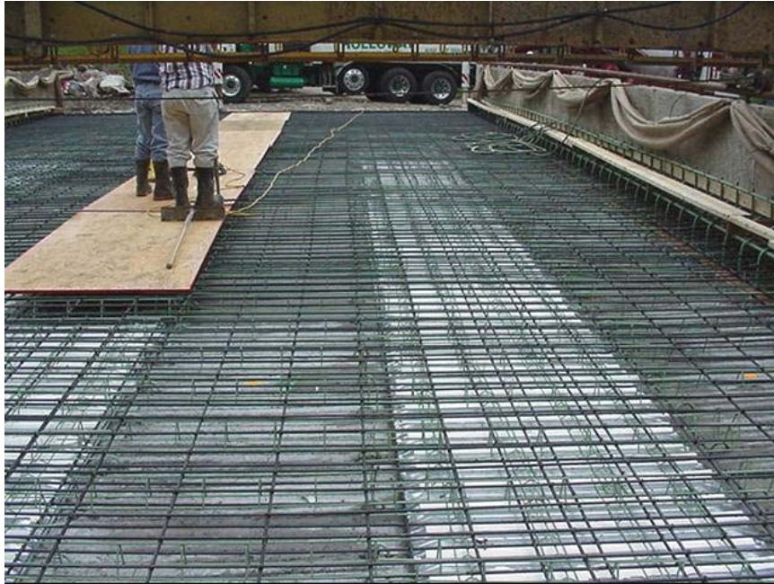
(a) Placement of CFRP bars
