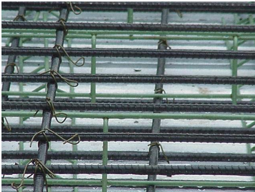
(b) Close-up view of CFRP bars
