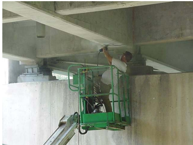
Fig. 3.1 – Preparing concrete substrate for CFRP laminates.
