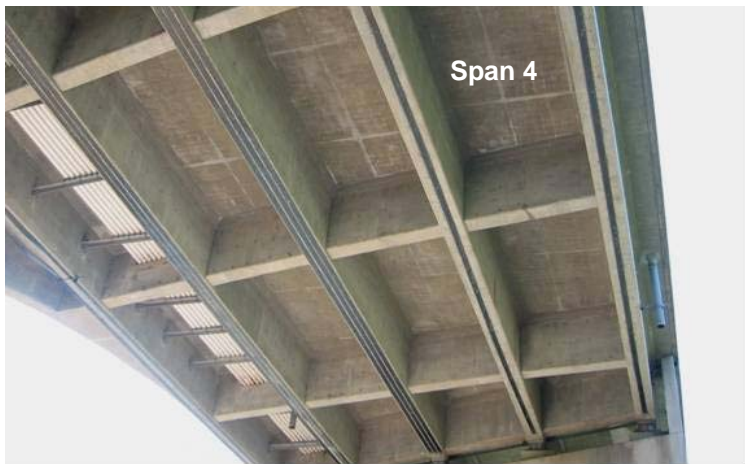
(b) Span 4 of the middle reinforced concrete span
