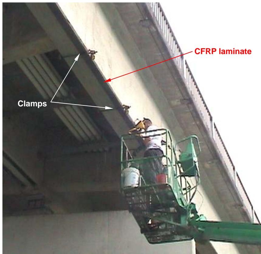
Fig. 3.2 – Application of CFRP laminate to RC girder.
