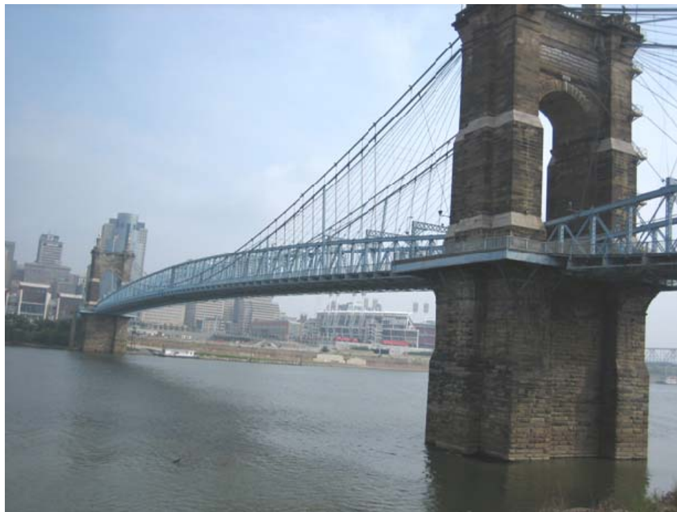
Fig. 1.1 – The John A. Roebling Bridge carries KY 17 over the Ohio River between Covington, KY, and Cincinnati, OH.
