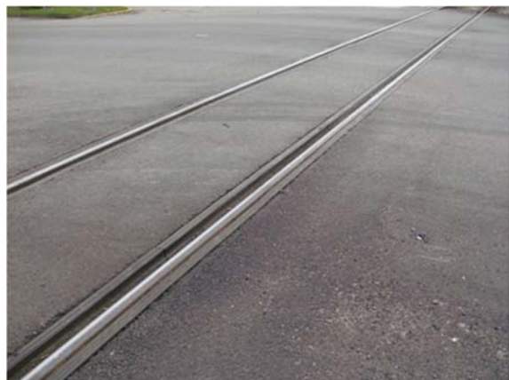
2011 – Converted to Rubber Seal/Asphalt in 2010
