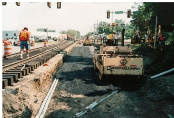
2005, Compacting the Asphalt Underlayment
