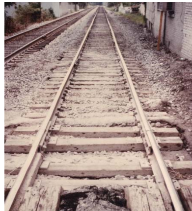
October, 1984 – Before Renewal
