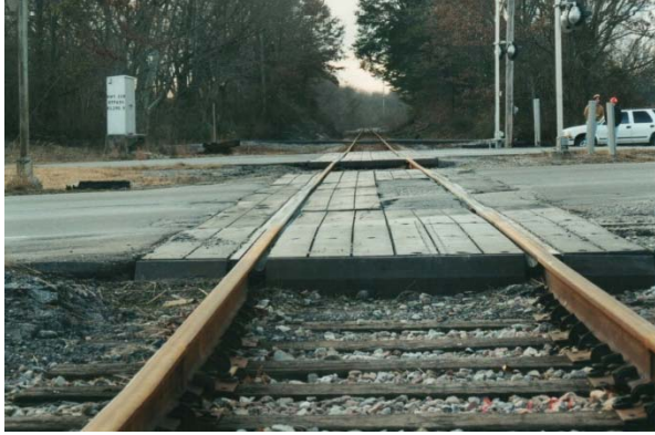
2001, Prior to Renewal, Note the Settlement of the Crossing
