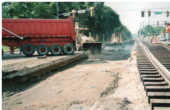
2005, Spreading the Asphalt Underlayment
