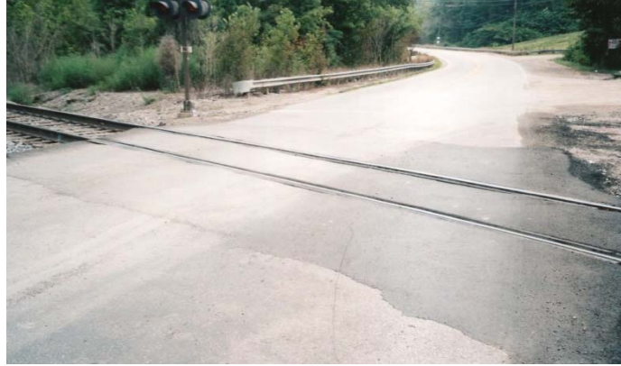
2006 After Renewal due to Derailment
