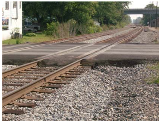
2013 After Replaced with Timber/Asphalt Surface Earlier in the Year
