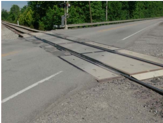
2013 After 11 Years of Service, Containing Numerous Asphalt Patches
