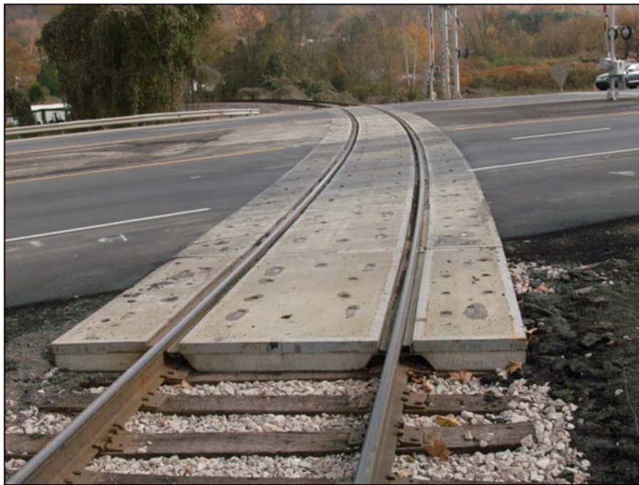
Figure 2.3. U.S. 25E – Barbourville, KY Concrete Panel Crossing Surface.
