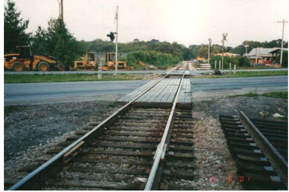
2001, Prior to Renewal, Note the Settlement of the Crossing
