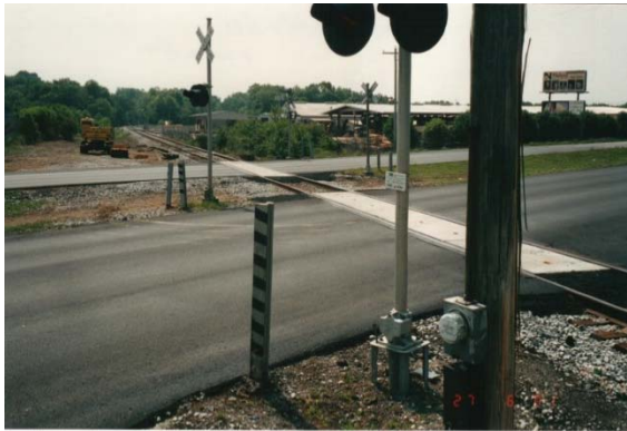
Finished Project, Two Weeks Later
