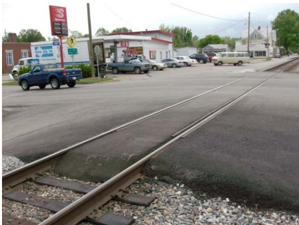
2011 – Converted to Rubber Seal/Asphalt in 2010
