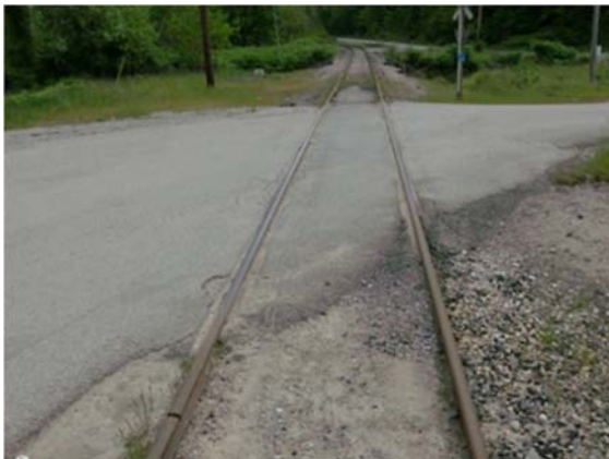
2013, Similar Condition, Slight Raveling of Flangeways
