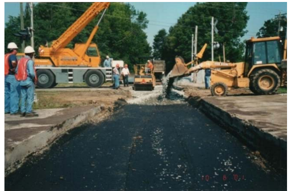
Rolling Ballast on Compacted Asphalt
