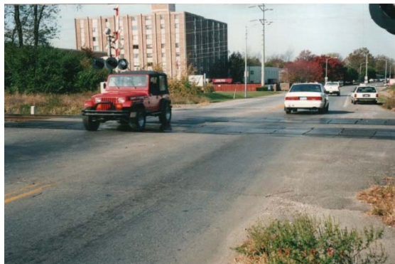
October, 2001- Before Renewal
