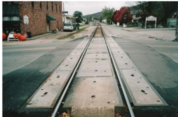
October 2006 After Surfacing/ Replacing Panels
