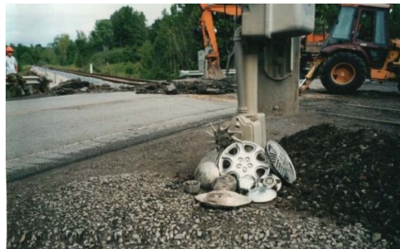
2002 Removing the Old Surface
