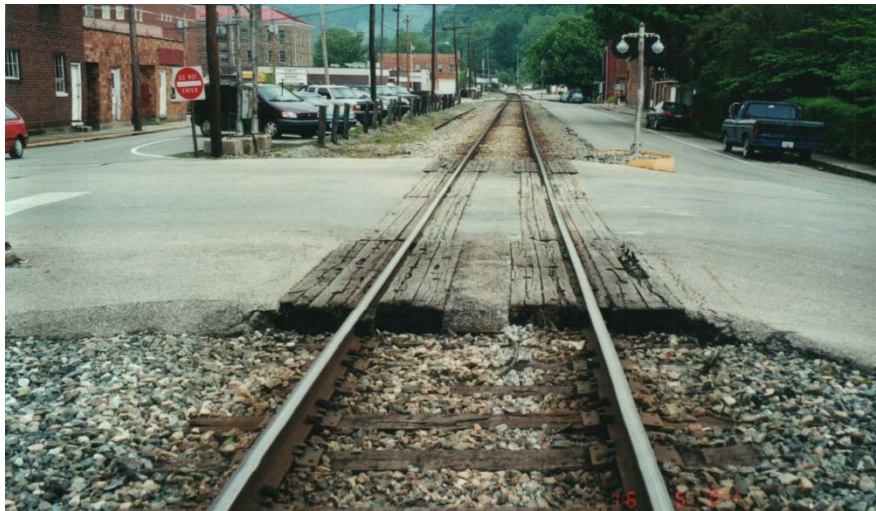
2002- Before Renewal with Concrete Surface
