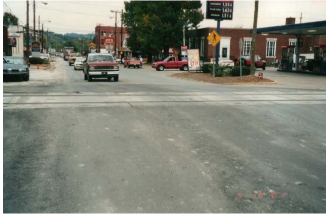
November 2001-After Renewal with Concrete
