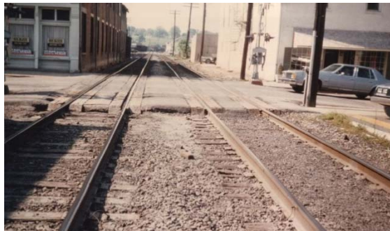
October, 1984 – Before Renewal
