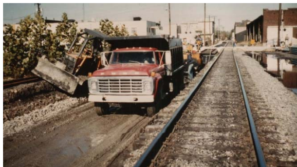
October, 1984 – During Paving
