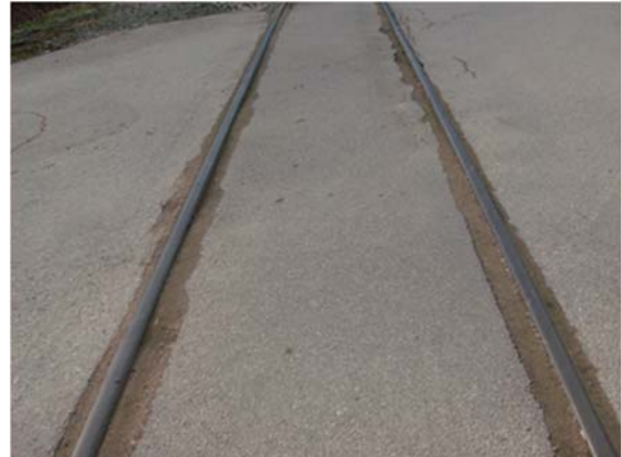
2013, Similar Condition, Slight Raveling of Flangeways
