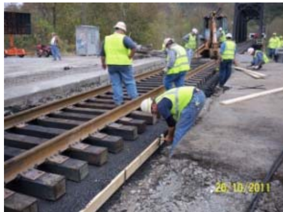
November 2011 During the Installation
