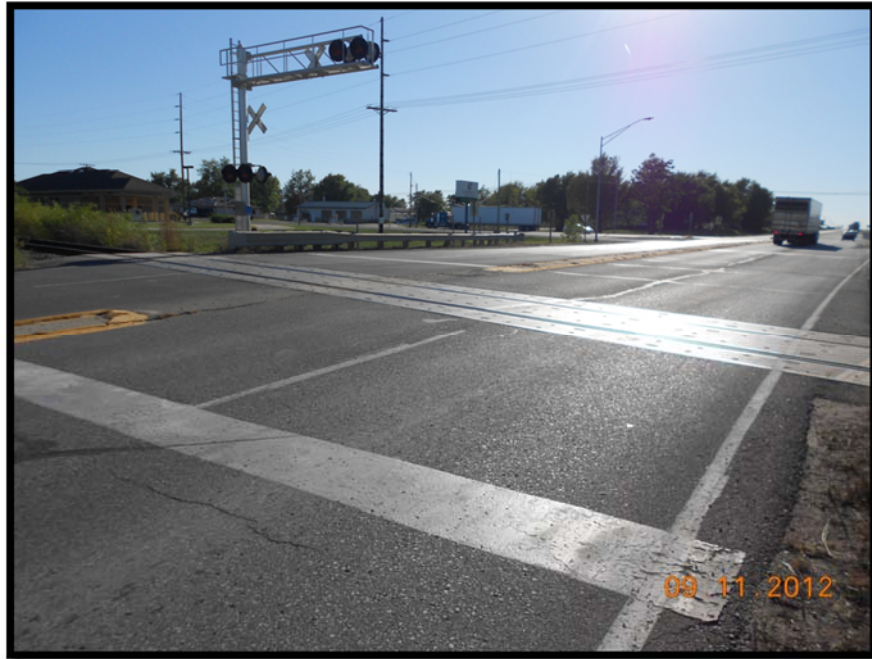
Figure 3.3. Albia, IA Crossing Underlain with Asphalt.
