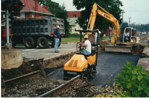
2000, Compacting the Asphalt Underlayment
