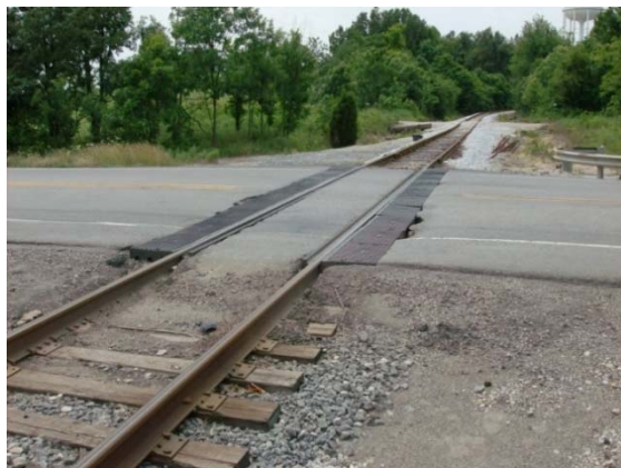
2011 Rubber Panels and Rail were Loose and Deflected Under Heavy Loads
