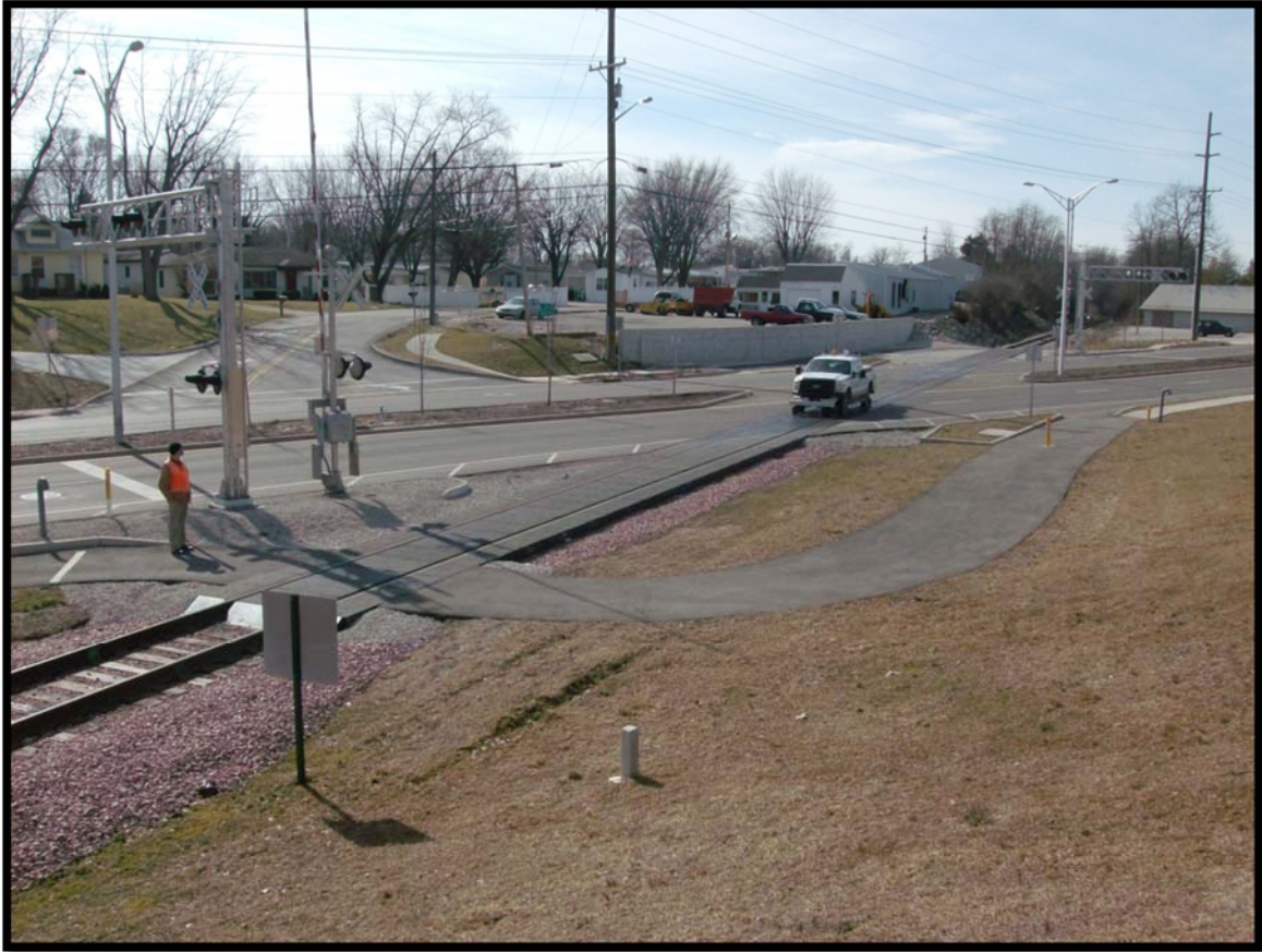
Figure 3.9. 3rd Street Crossing on the INRD in Bloomington, IN, Underlain with Asphalt.
