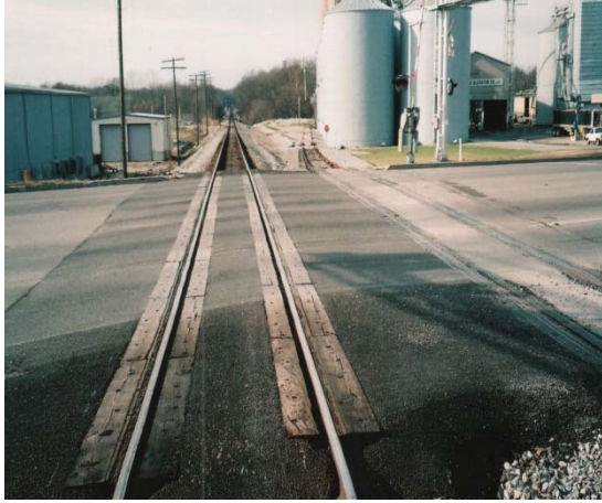
2006, Main Track Immediately After Renewal 2006, Industry Spur Track, not Renewed in 2006
