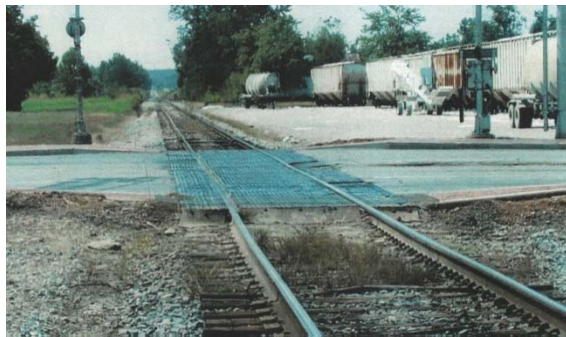
2009- Mainline Before Renewal
