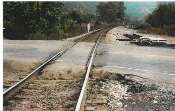
October, 2001 – Before Renewal
