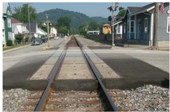
2013, After Removing Panels, Surfacing Through, and Repaving Approaches
