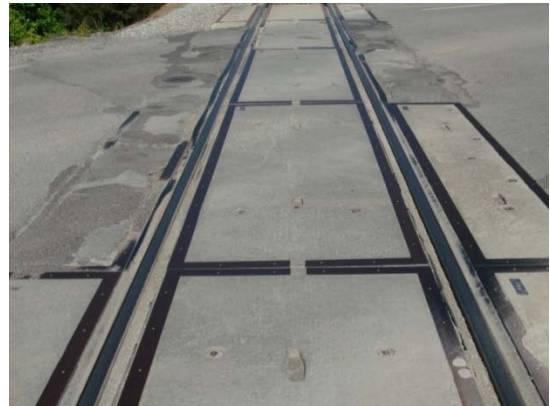
2013 After 11 Years of Service, Containing Numerous Asphalt Patches
