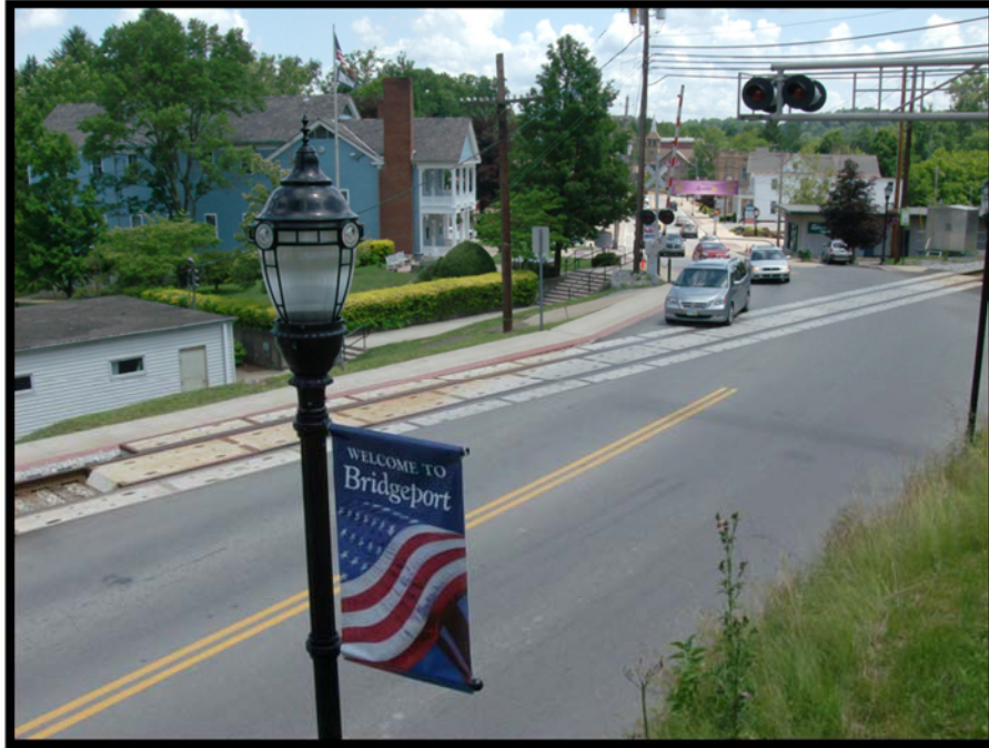
Figure 3.4. Bridgeport, WV Crossing Underlain with Asphalt.
