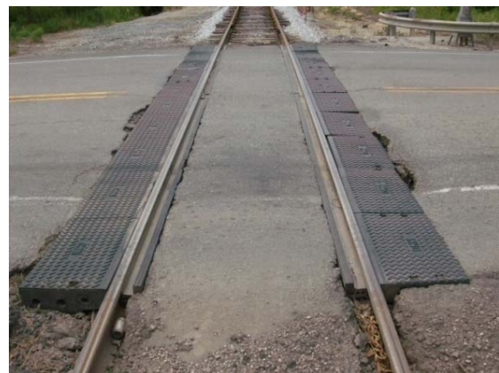
2011 Rubber Panels and Rail were Loose and Deflected Under Heavy Loads
