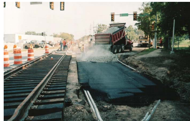
2005, Dumping the Ballast on the Underlayment
