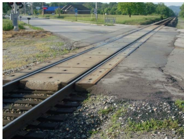
2011 After Replacing Rail and Reusing Surface
