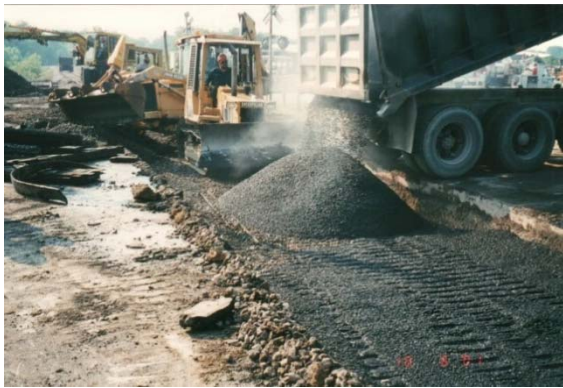
Dumping & Spreading Asphalt Underlayment
