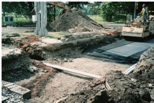
2005, Compacting the Second Lift
