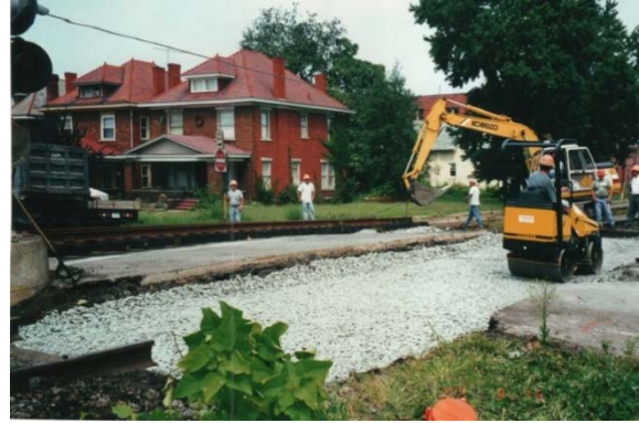
2000, Compacting the Ballast
