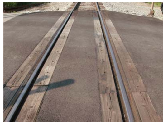
2013 After Renewing with Timber/Asphalt Surface Earlier in the Year
