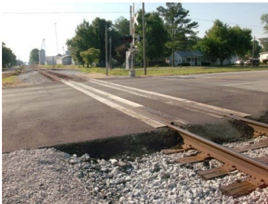
2013 Timber/Asphalt Surface Placed in 2012 During Timbering Program
