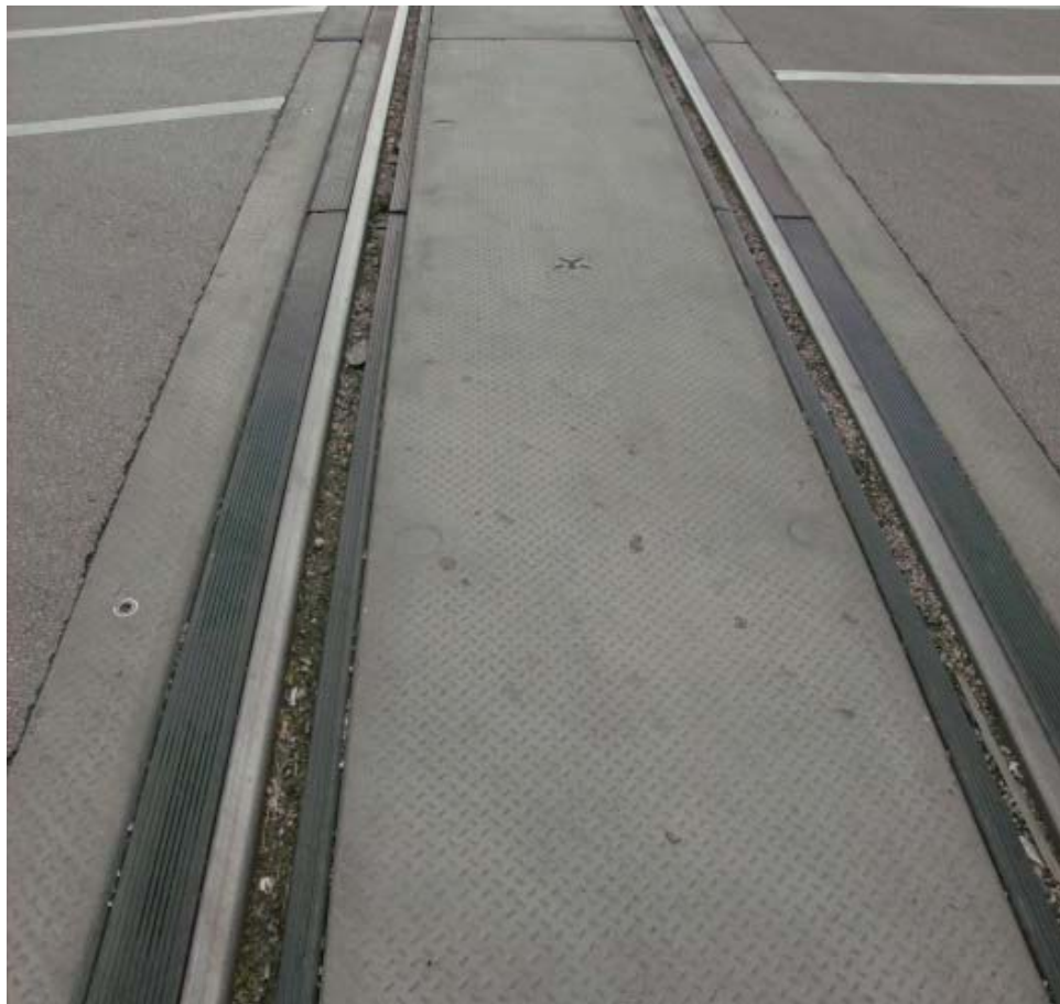
Figure 3.6. Concrete Tub Crossing in Urbana, IL.
