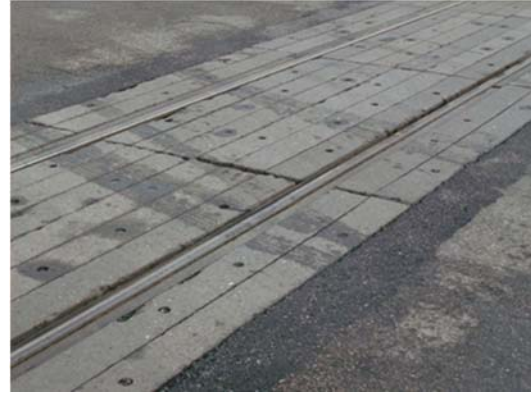
2011 After Changing out Rail and Replacing Composite Surface. Still in Perfect Condition
