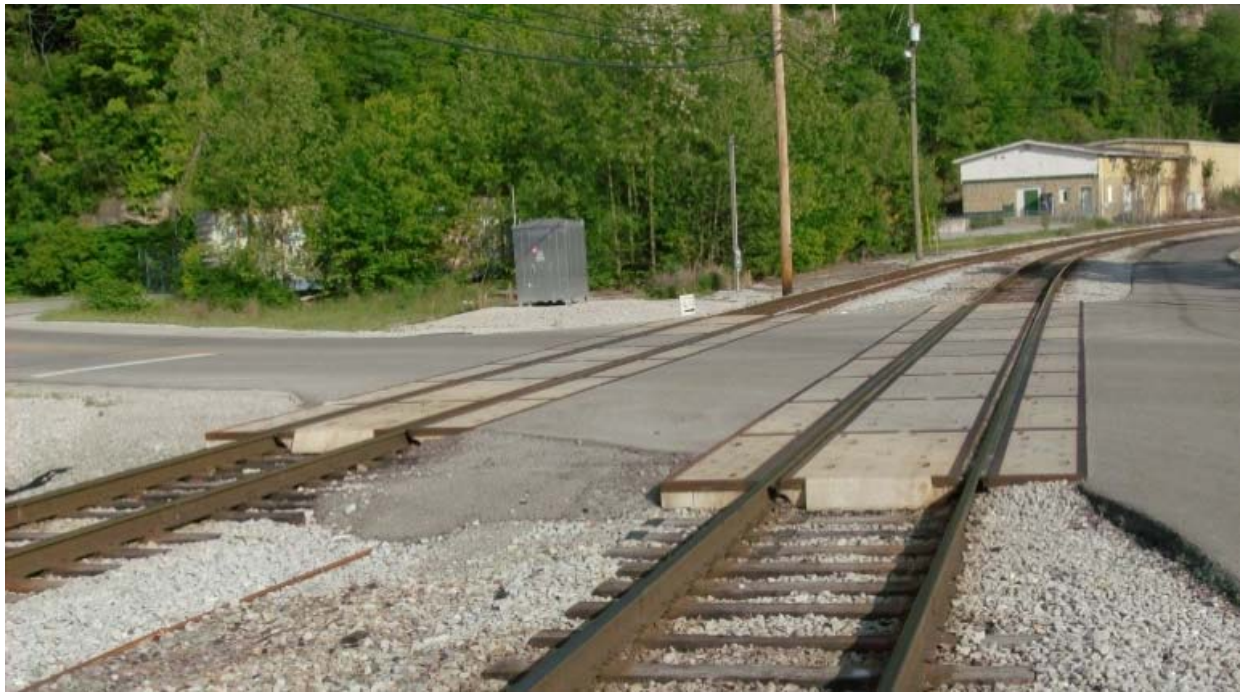
Typical Concrete Panel Crossing Surface
