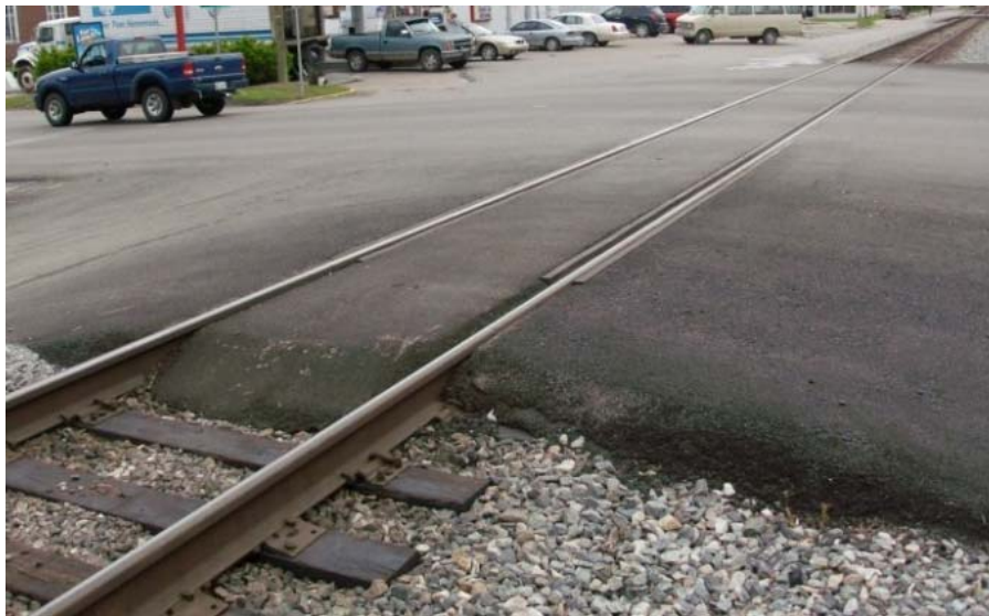
Typical Rubber/Asphalt Crossing Surface
