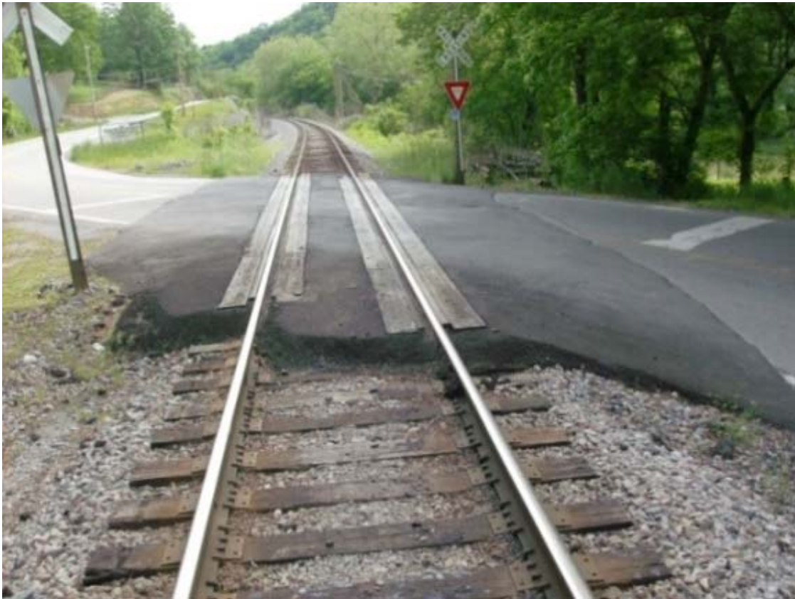
Typical Timber/Asphalt Crossing Surface
