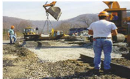
Positioning new panel
