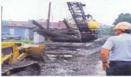
Lifting out old Panel
