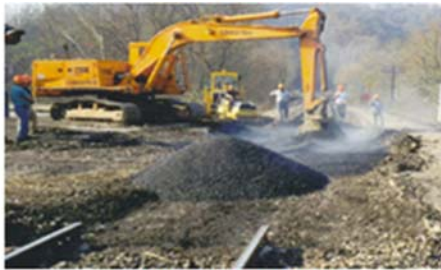
Spreading asphalt
