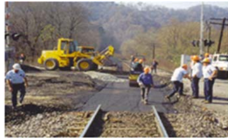
Compacting asphalt and dumping ballast
