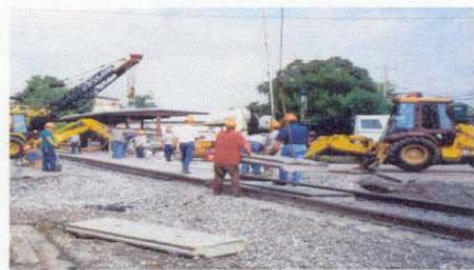
Placing concrete surface
