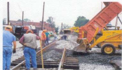
Dumping cribbing rock
