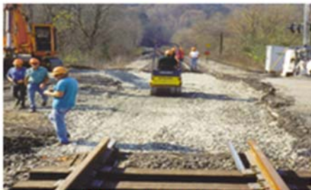
Compacting ballast
