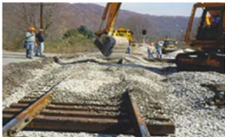
Spreading cribbing rock
