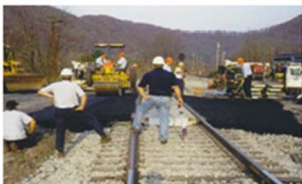
Compacting hand-spread approaches
