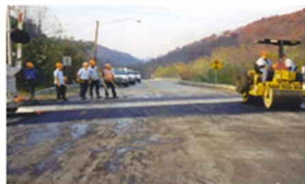
Finished compacting asphalt approaches
