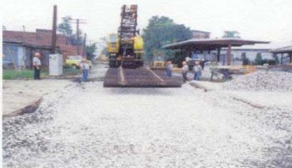
Positioning wood tie panel
