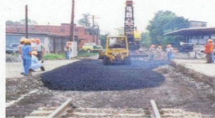
Compacting placement of asphalt
