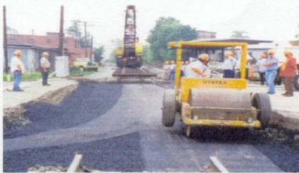
Compacting asphalt
