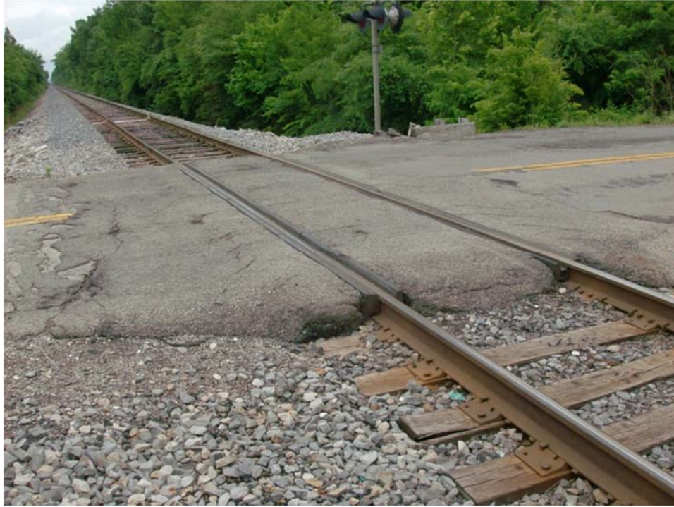
Figure 3.4. No settlement, rough approaches.
