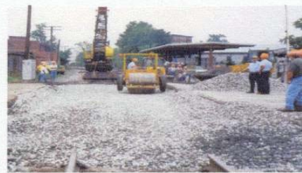
Compacting ballast
