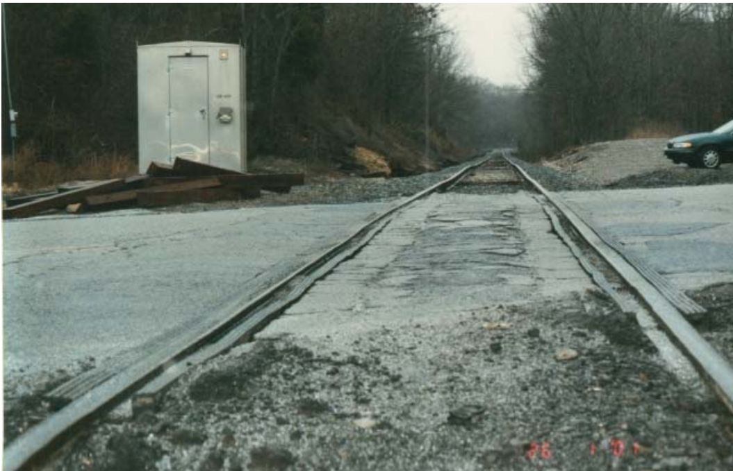
Figure 3.8. Deteriorated surface.
