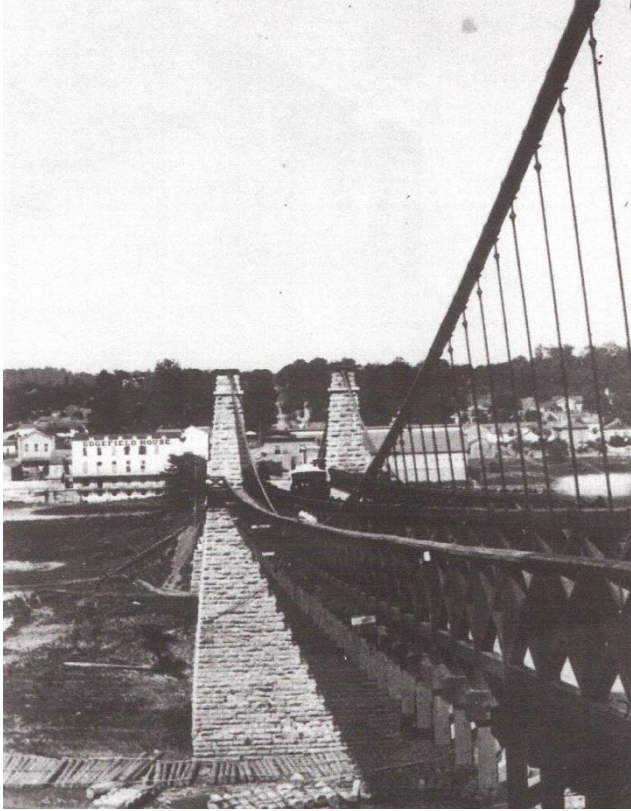
Figure 2.1. Opening of the Woodland Street Bridge. 5
