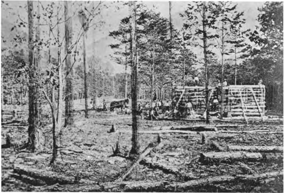
Erection of a log house, showing cornermen and facilities for lifting logs into position
