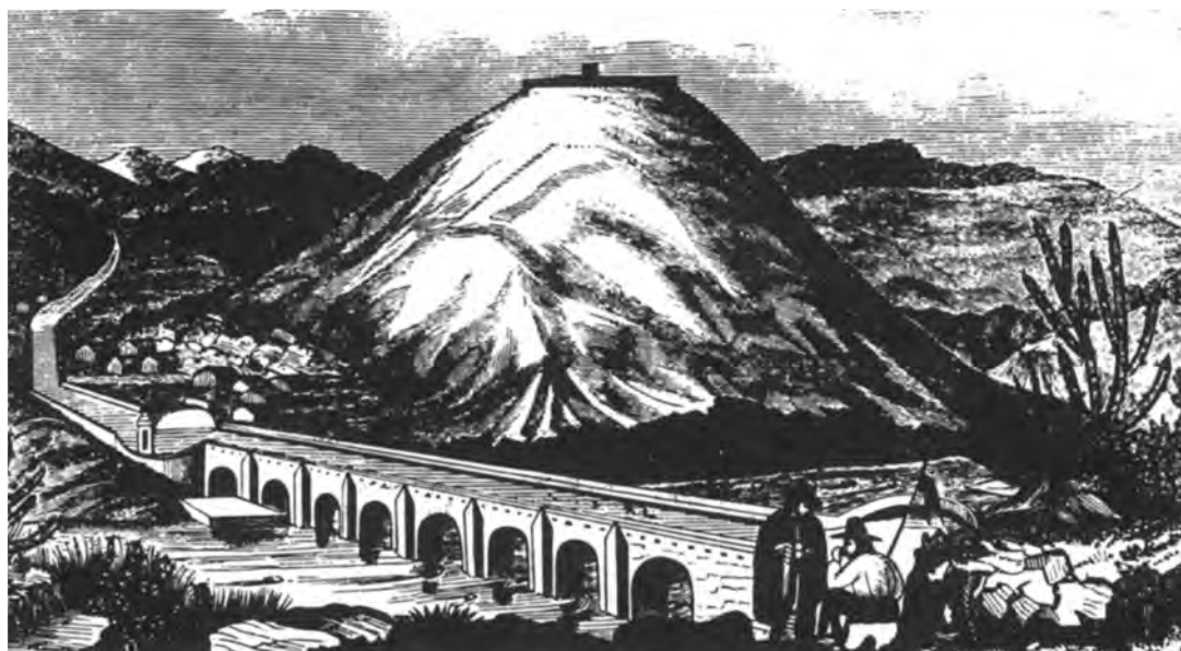
The National Bridge from the bluffs on the east.
