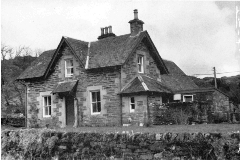
22 Schoolhouse at Ford, with the school attached at the rear. It has been used as a private residence since the school closed in the 1970s. (JBS)
