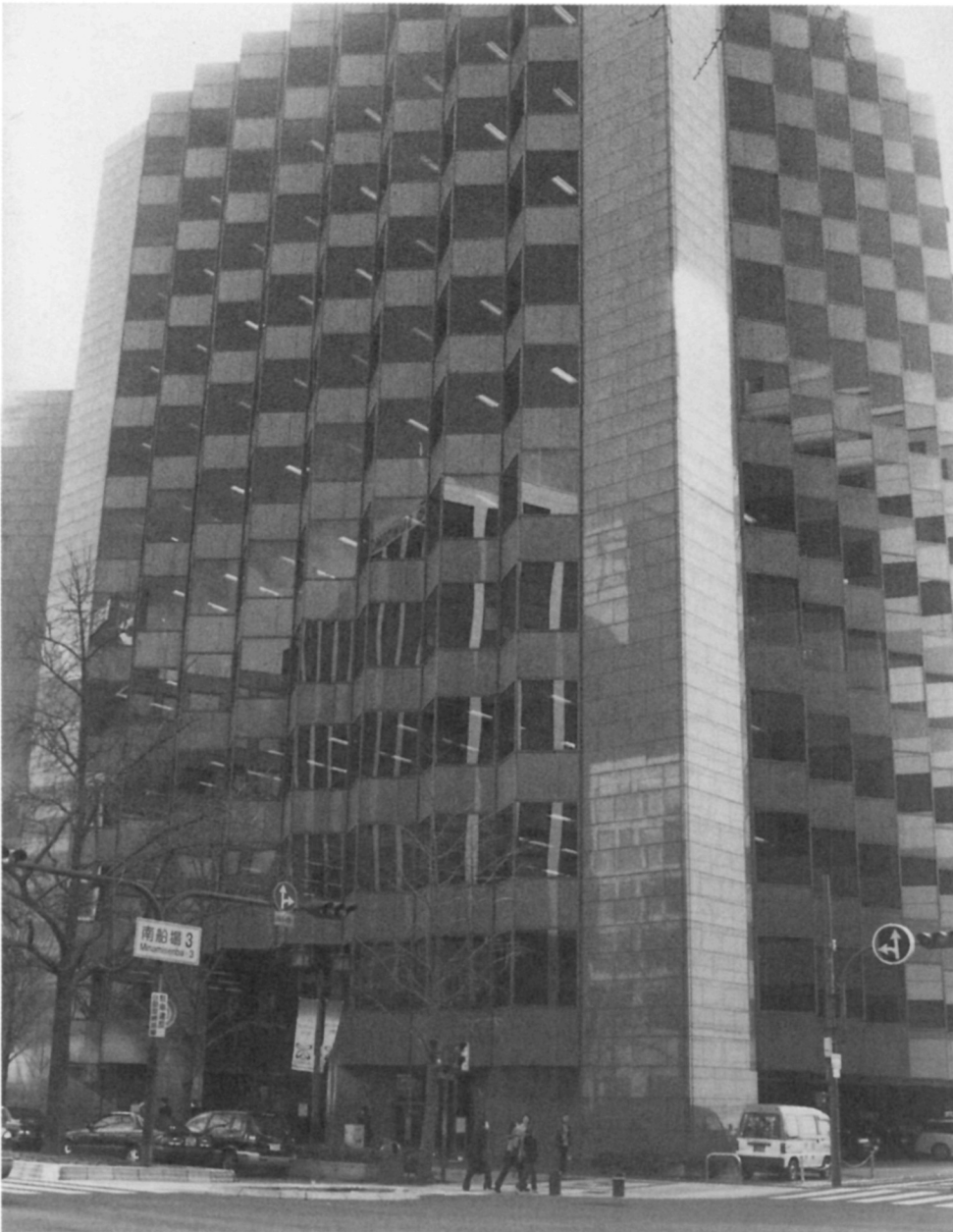
The headquarters of Matsushita Corporation in Minami Senba area of Osaka, Japan. Matsushita operates plants in Danville and Berea, Kentucky. The quality of its engineering and the efficiency of its mass production techniques are second to none. Japanese companies such as Matsushita are going abroad to get away from Japan's high costs. Matsushita, for example, doubled its overseas workforce between 1992 and 1999 to 134,000, but took only 6,000 new people in Japan. Over the same period, Hitachi, which has a plant in Harrodsburg, Kentucky, also nearly doubled its number of overseas employees, but reduced its workforce in Japan by 3 percent to 267,000. (Photograph by P.P. Karan)
