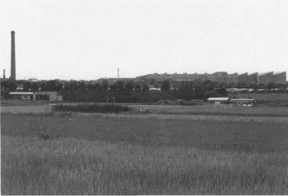
Toyota's Takaoka Plant in the southwestern part of Toyota City, Japan, lies in the midst of rice fields. The plant started operations in 1966 and has plastic molding, stamping, body, painting, and assembly shops. It produces Prius, Corolla, Sprinter, Tercel, and Paseo passenger cars. (Photograph by Yuichiro Nishimura)
