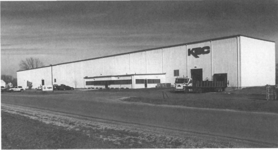
Kentucky Steel Center, located in an industrial park in Berea, Kentucky, was established in 1996. The plant processes steel and is wholly owned by Sumikin Bussan Corporation of Osaka, Japan. (Photograph by P.P. Karan)
