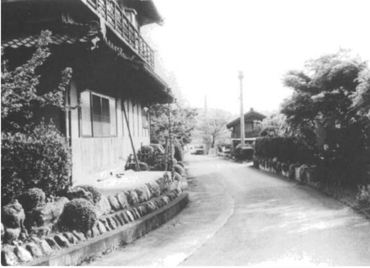
61. A prefectural road, with no shoulders, in the northwestern part of the Kanto Plain, Honshu—an area designed before the advent of automobiles. This road is a thoroughfare for pedestrians, bicyclists and motorists. Japan had 80,173 miles of prefectural roads and 583,744 miles of local roads in 1991. Virtually all roads are paved. The total expenditure in 1990 on roads was $65.2 billion or approximately 3.2 percent of the gross national product.
