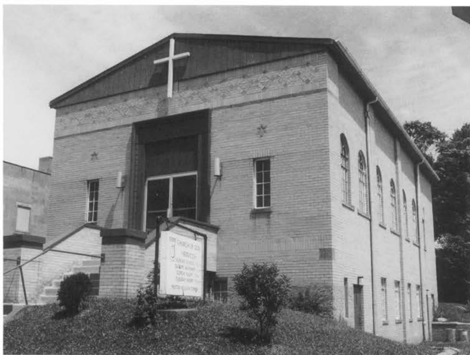
Figure 77. The Temple of Israel building in Covington as it looked in the early 1990s. The roof line has been changed completely, and little evidence remains that it was once a synagogue (compare Figure 41).
