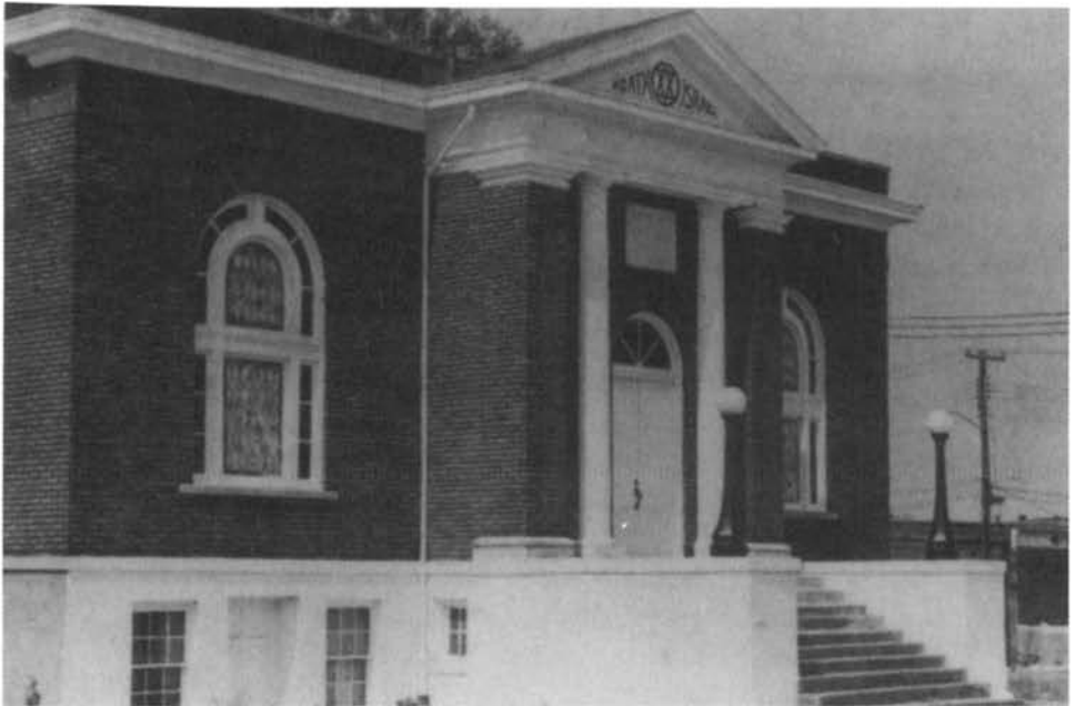
Figure 39. Adath Israel, Sixth Street, Hopkinsville. This building, constructed in 1925, was demolished in 1977 after its roof collapsed under a heavy snow. From William T. Turner, comp., A Pictorial History of Hopkinsville and Christian County since 1865 , vol. 2 of Gate Way from the Past (Hopkinsville, Ky., 1974).
