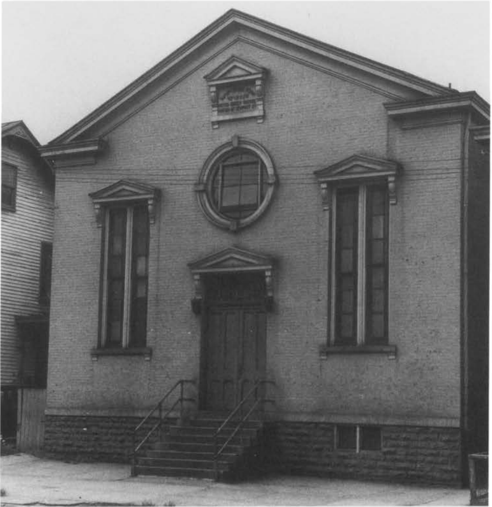
Figure 27. United Hebrew Congregation, Fifth Street, Newport. Originally a church, this building served as an Orthodox synagogue for more than six decades and then became a church again. This picture was taken around 1940. Photograph by Myron Benson, courtesy of the Bureau of Jewish Education, Cincinnati, Ohio.
