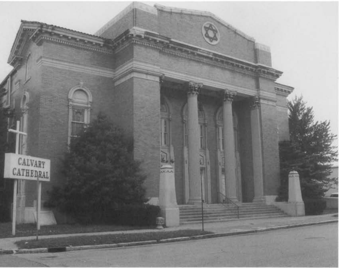
Figure 44. The Keneseth Israel building, Jacob Street, Louisville, as it appeared in the early 1990s. Like the other two synagogue buildings still standing in downtown Louisville, it is on the National Register of Historic Places and now serves as a church.
