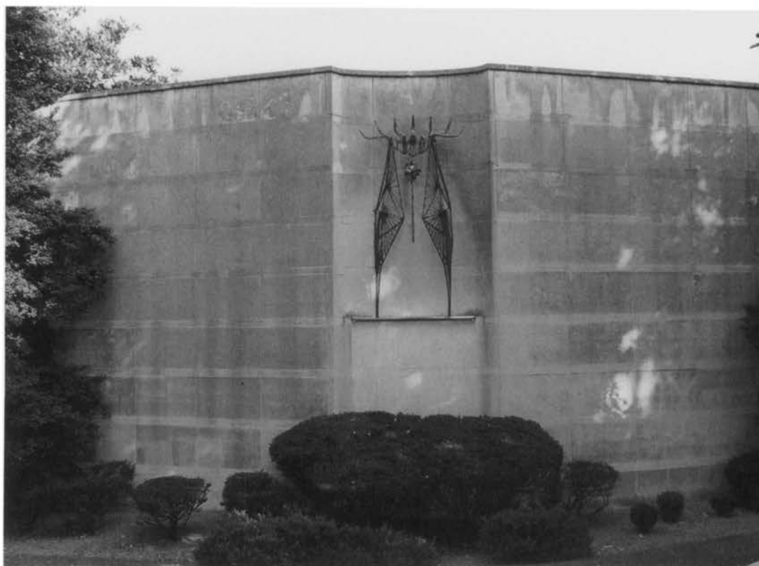
Figure 76. The controversial sculpture by Henry Roth on the facade of the 1957 Adath Jeshurun synagogue in Louisville.
