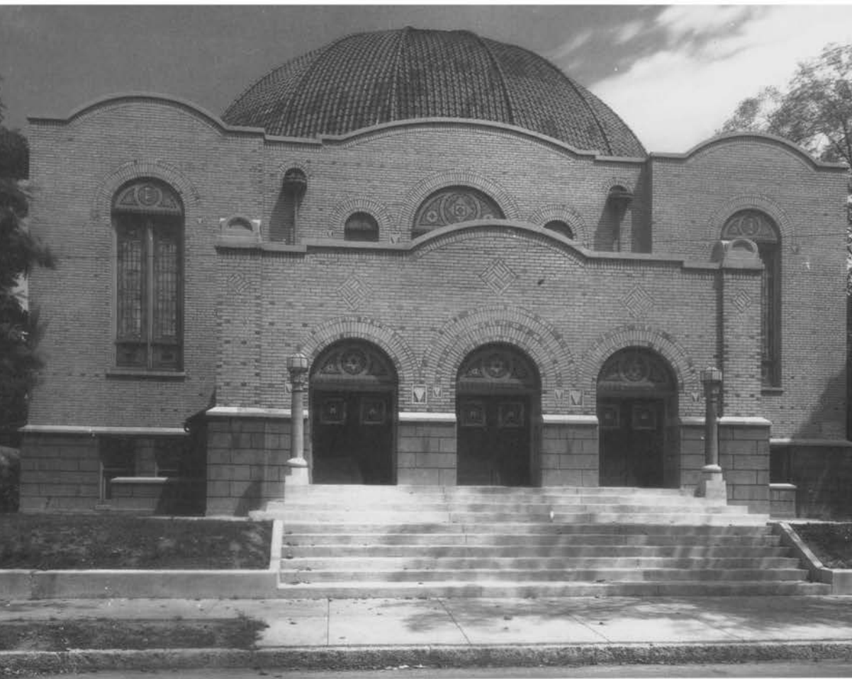
Figure 37. Adath Jeshurun, Brook Street, Louisville. This Byzantine style structure was erected in 1919 and served Adath Jeshurun until 1957. From the University of Louisville Photographic Archives, Caufield and Shook Collection (neg. 37570).
