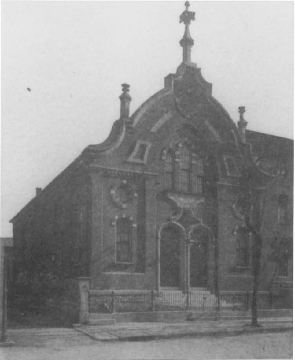
Figure 22. Brith Sholom, First Street, Louisville. This 1881 building, whose original facade is known today only from this poor-quality newsprint image, underwent substantial alterations after it passed to the Anshe Sfard congregation (see Figure 43). From History of the Jews of Louisville, Ky. (New Orleans, 1901).
