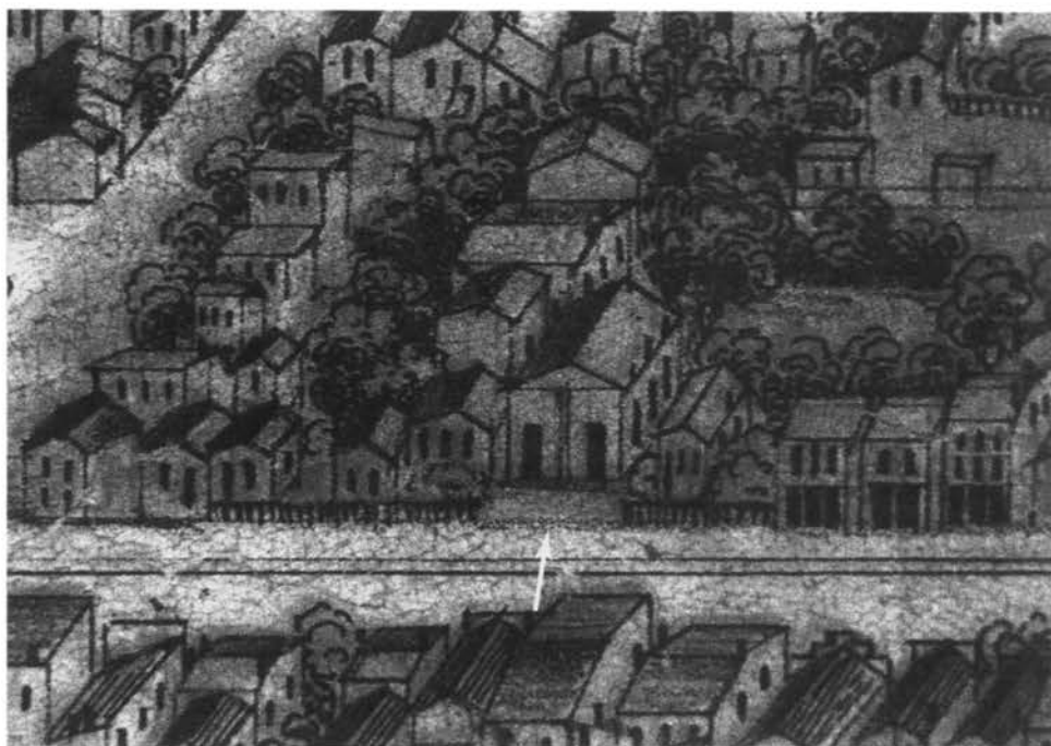
Figure 24. B'nai Jacob, Jefferson Street, Louisville. This church (indicated by the arrow) was occupied by the B'nai Jacob congregation in the last decade of the nineteenth century and then replaced by a new building on the same site (see Figure 34). The church is shown here in J.T. Palmatary's 1855 bird's-eye-view map of Louisville. Photo by Tom Fougousse.
