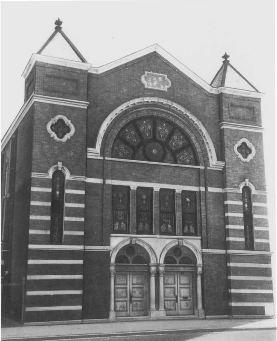
Figure 34. B'nai Jacob, Jefferson Street, Louisville. This building was dedicated in 1901 on the site of a former church that had served as B'nai Jacob's synagogue from 1891 (see Figure 24). Photo courtesy of Keneseth Israel Congregation.
