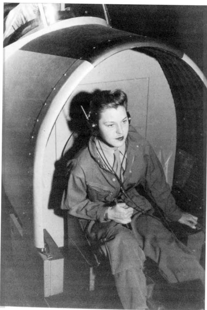
WAC private Betty S. Dayton working with a U.S. Military Academy cadet in the "Gunairinstructor." As the gunnery instructor, Private First Class Dayton would fly the enemy airplane on a projection screen and teach the cadet how to shoot down his target. Photo from U.S. National Archives and Records Administration, Still Pictures Branch (342-FH-4A-05169-119416AC).
