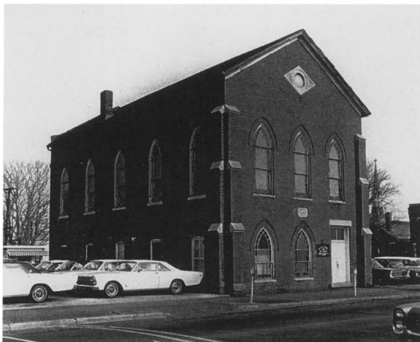
Evansville's Alexander Chapel African Methodist Episcopal Church, located near Fifth and Walnut Streets. This edifice, which the congregation built in 1889, stood until the advent of urban renewal during the 1960s. Courtesy Special Collections, University of Southern Indiana, Evansville
