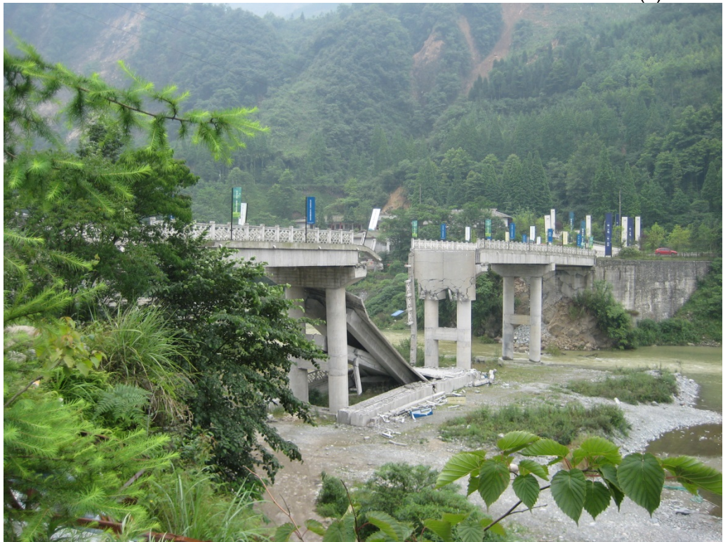
Figure 2.6: Bridge Damage from the 12 May 2008 Wenchuan Earthquake. Examples of damage to bridges in the Wenchuan, China, area caused by the 12 May 2008 Wenchuan earthquake. Photos: ©Zhenming Wang 2008.
