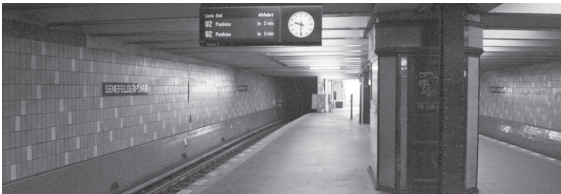
fig 4.04 Maintenance closet and northbound platform at Senefelderplatz
