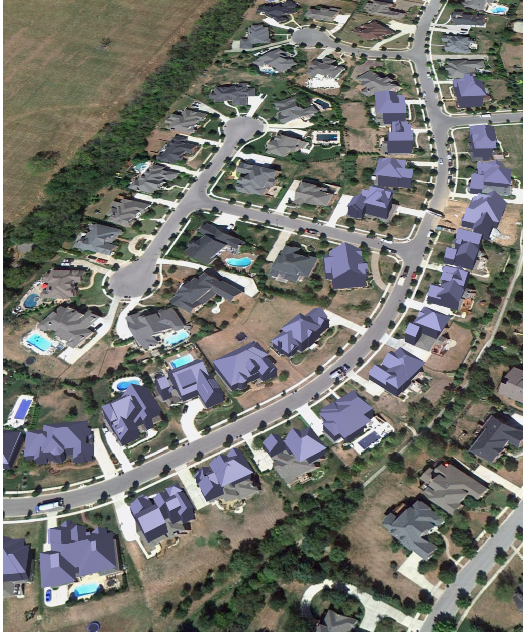
Figure 5.18: An overall view of reconstructed houses in Div-A.
