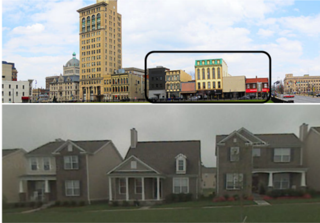
Figure 5.4: Examples of independent buildings that we aim to segment. Top: a downtown area. Bottom: houses in a suburban area. Notice that, we do not aim to segment the connected sub-facades in the black box.
