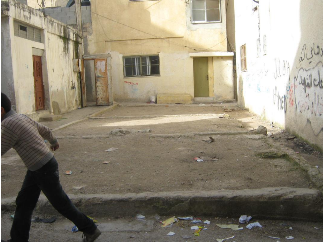
Figure 26. The destroyed home.
