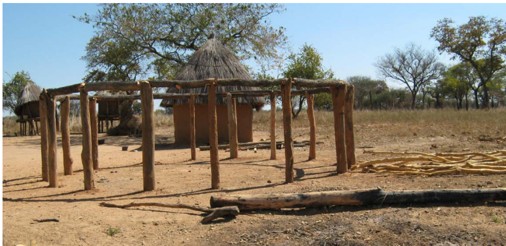
IMAGE 4.1: An example of a structure—a gathering shelter— under construction
