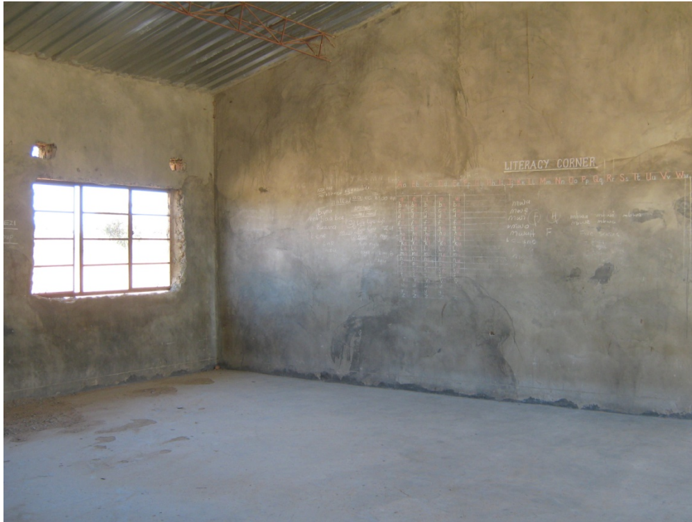
IMAGE 1.3: Inside the new schoolhouse at Inzoka Middle Basic
