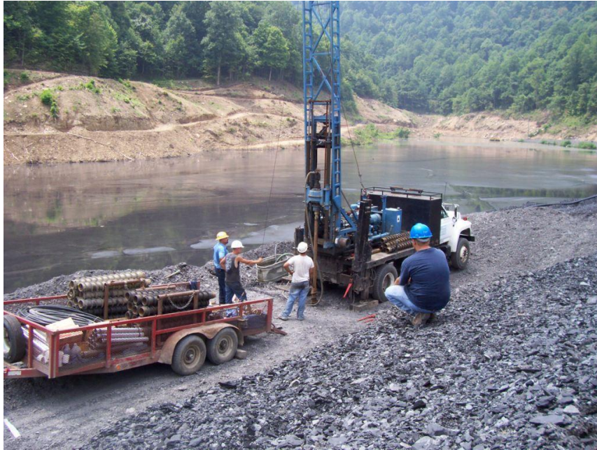
Figure 2.12: Performing drilling, SPT testing, and fixed piston sampling at Big Branch.
