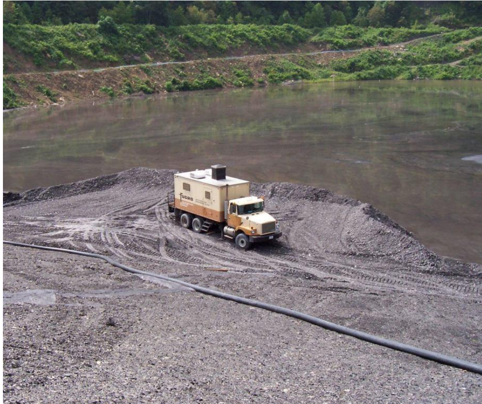
Figure 3.2: Constructed beach in the slurry pool.
