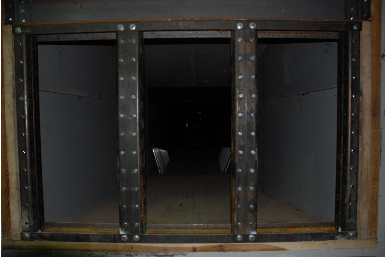
Figure 3.6. Steel Framing Bolted in Place
