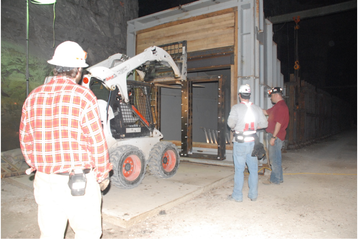
Figure 3.5. Steel Framing Final Placement for Bolting
