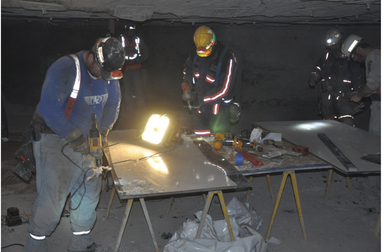
Figure 4.6. Cutting and Drilling Polycarbonate Panels
