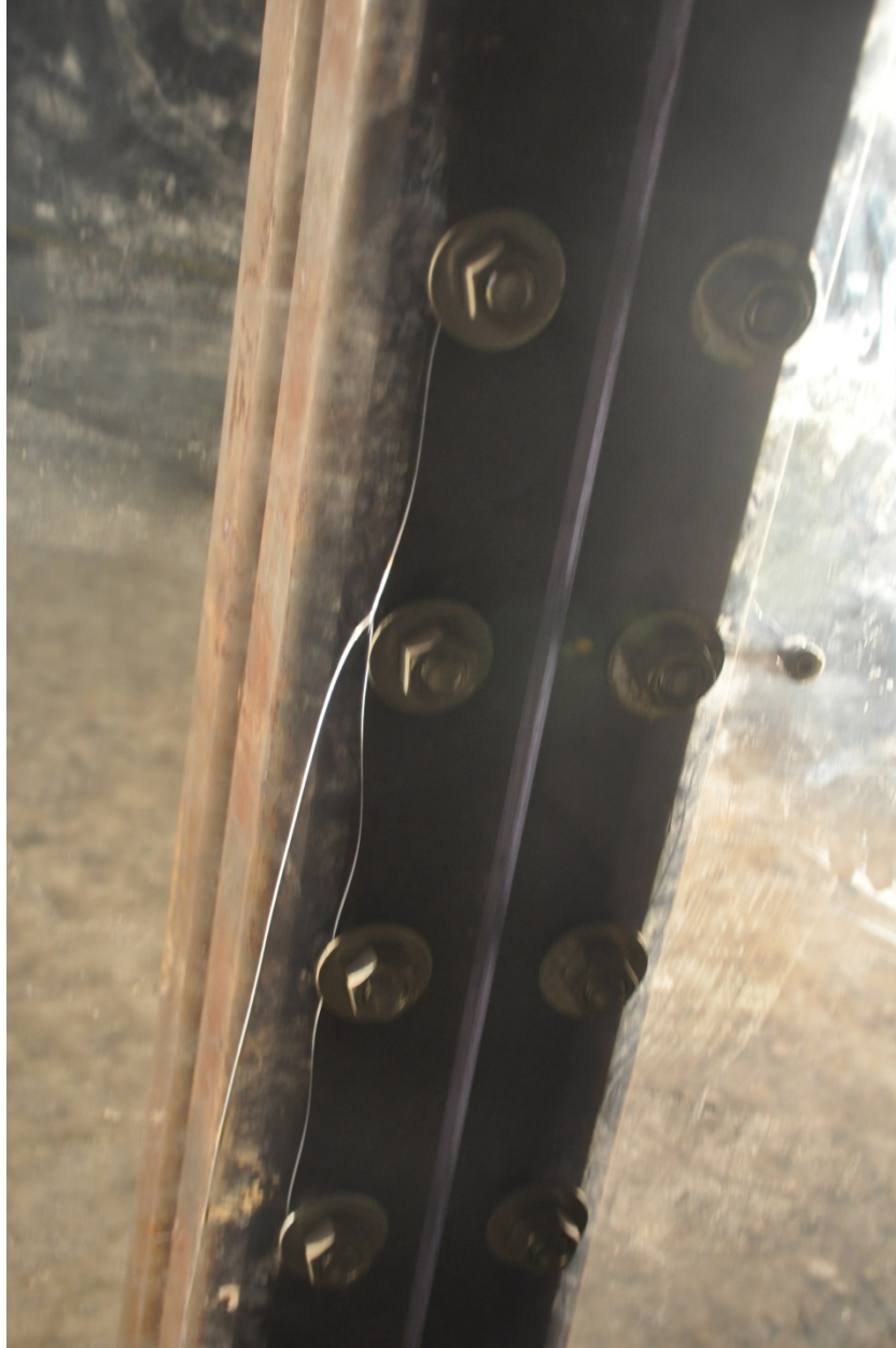
Figure 3.25. Crack in Polycarbonate Following Final Test
