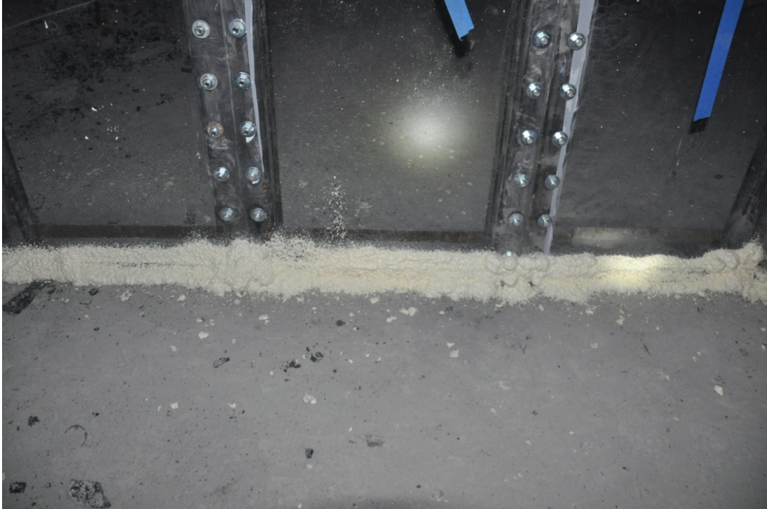
Figure 4.10. Mine Foam Sealing the Space between the Frame and Floor
