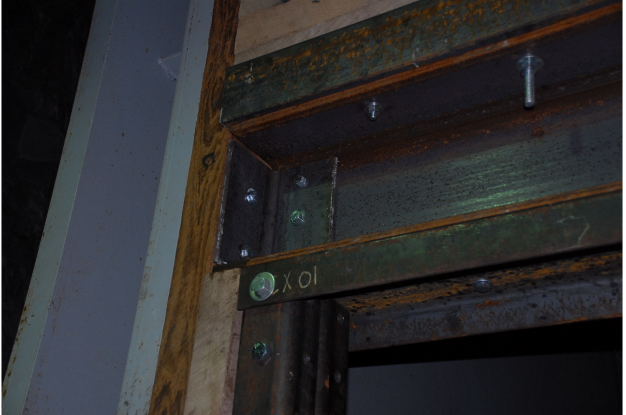
Figure 3.2. I-beam Horizontally Bolted Through Oak Boards to Steel Shock Tube Frame with Steel Angle
