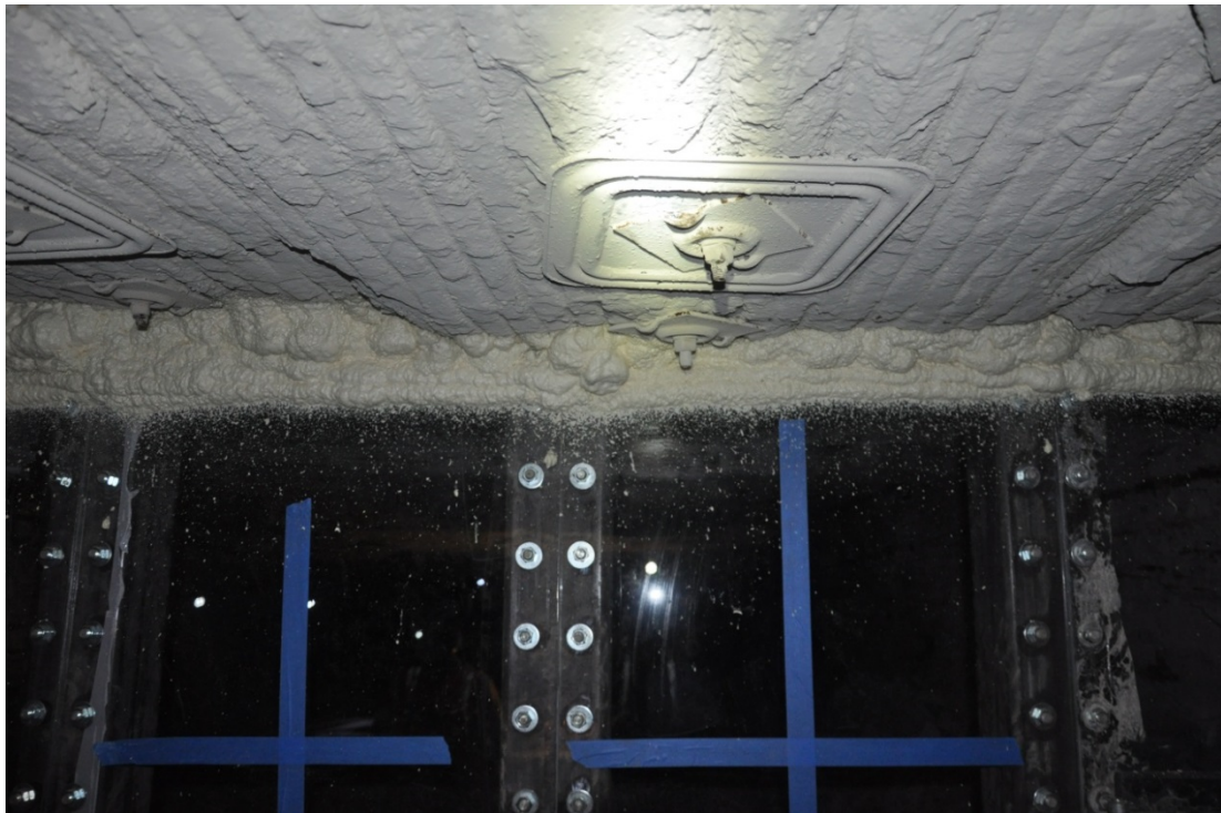
Figure 4.11. Mine Foam Sealing the Space between the Frame and Polycarbonate and
