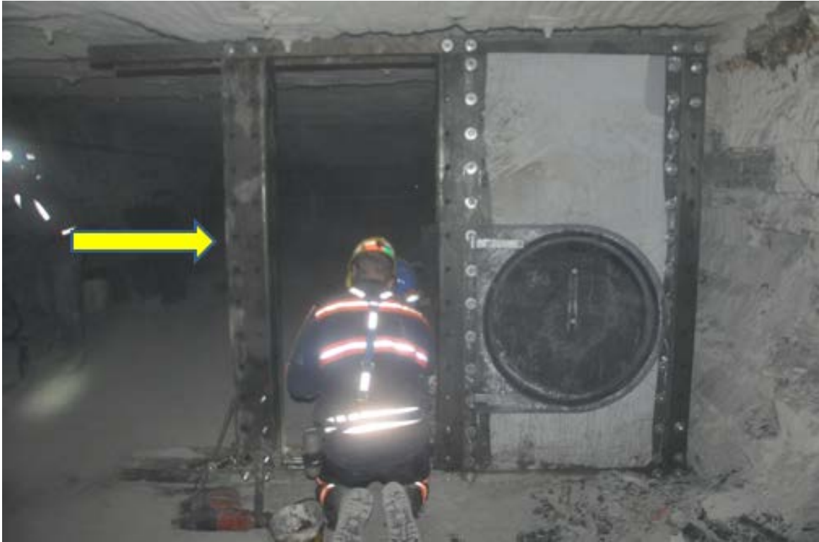
Figure 4.3. Second Vertical Support Installed
