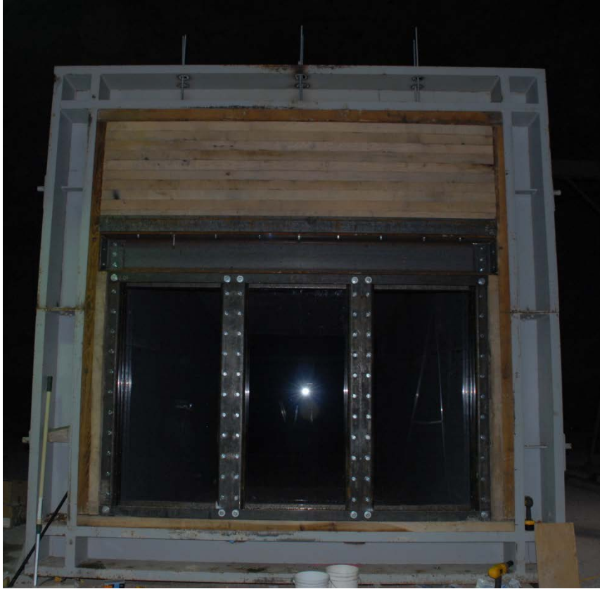
Figure 3.10. All Polycarbonate Panels Installed
