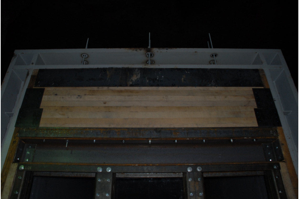
Figure 3.13. Steel Plate Placement on Outby Side of System
