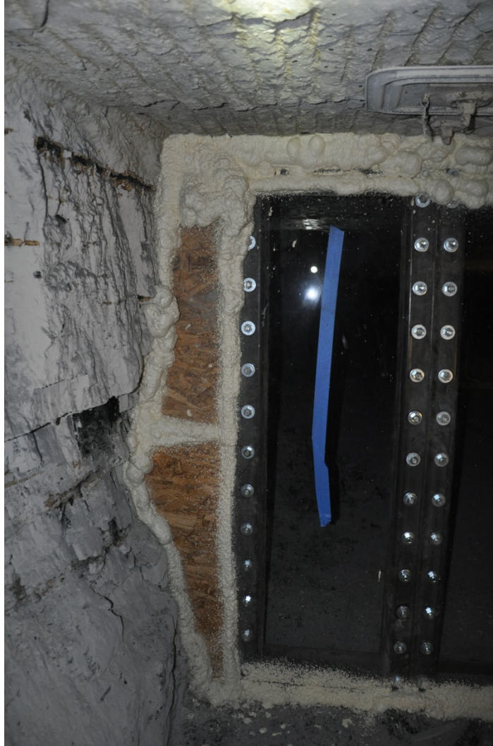
Figure 4.9. Plywood and Mine Foam Used to Help Seal the Wall
