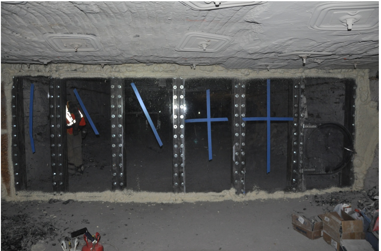
Figure 4.12. Final Sealed Installation Outside
