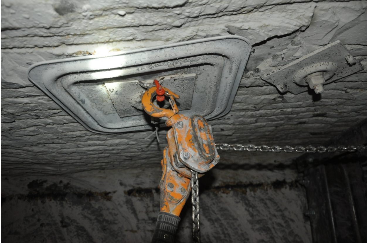
Figure 4.1. Chain Hoist Clipped in a Clevis Hooked into a Roof Bolt
