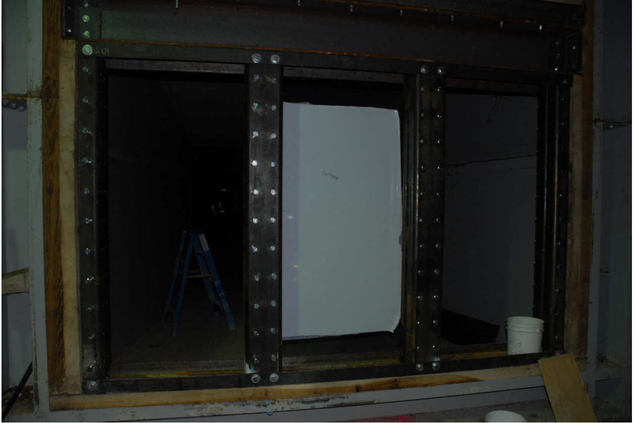
Figure 3.8. Middle Polycarbonate Panel Installation
