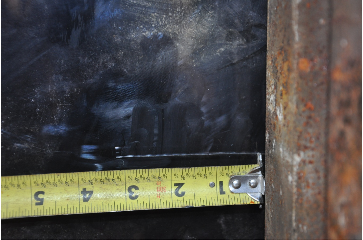
Figure 3.26. Crack from Previous Testing
