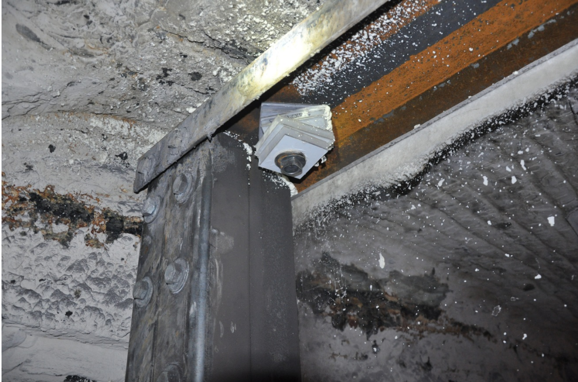
Figure 5.3. Polycarbonate Washers used on Hilti Bolts
