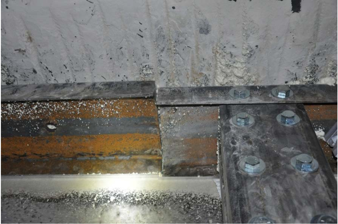
Figure 5.1. Intersection of the Top Two Channel Sections
