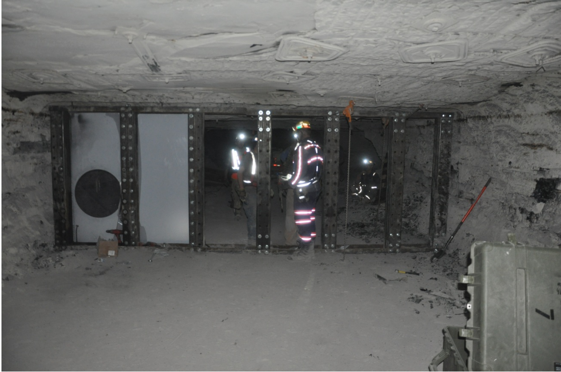
Figure 4.5. Completed Framing Installation
