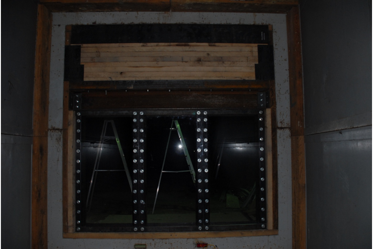
Figure 3.11. Steel Plate Placement on Inby Side of System
