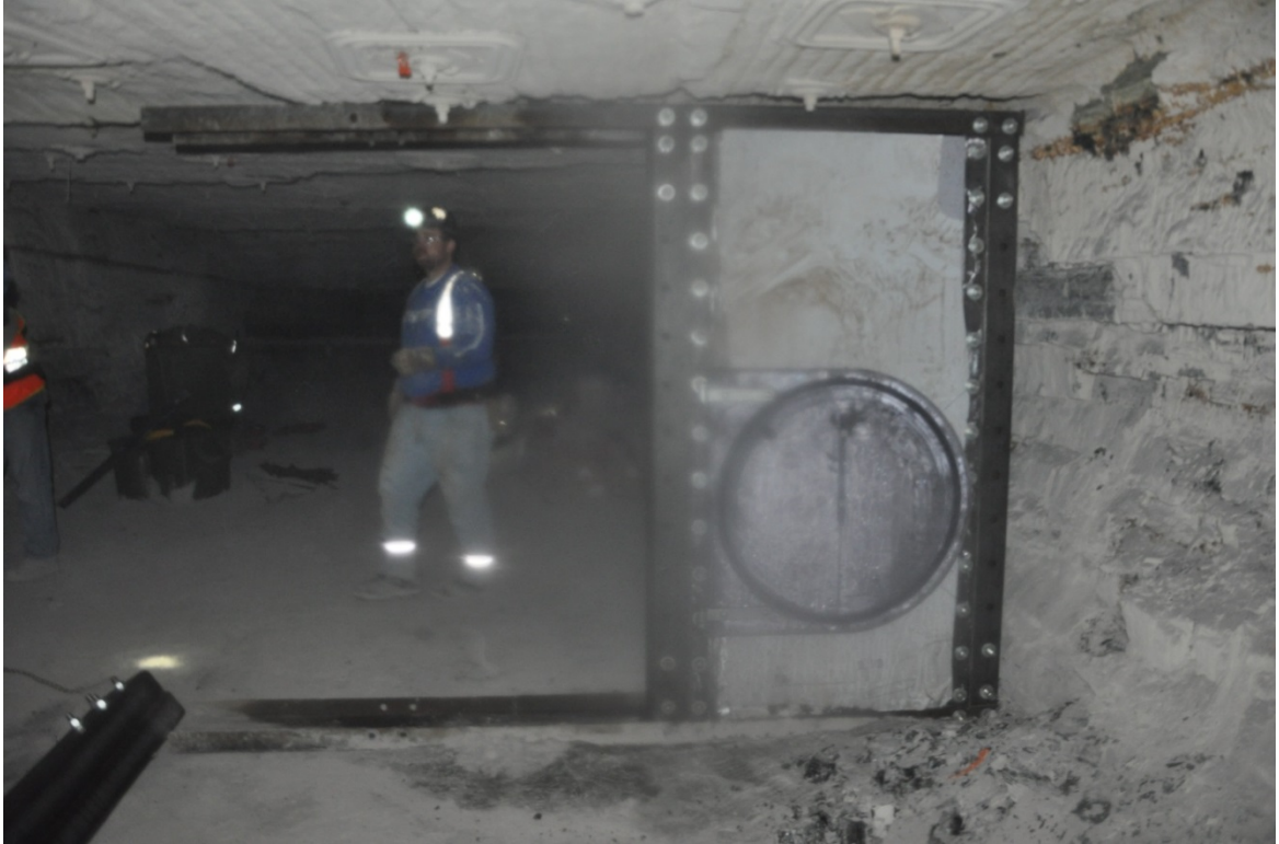
Figure 4.2. Installed Preassembled Door and Shorter Channel Section
