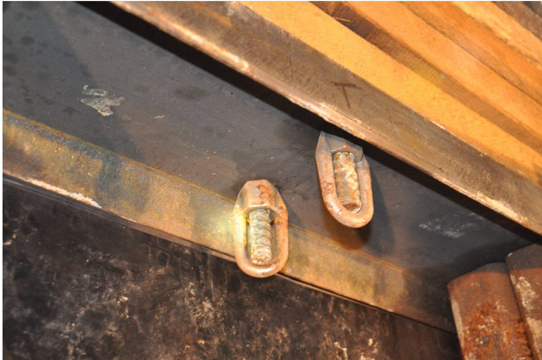
Figure 3.20. Roof Bolts Installed
