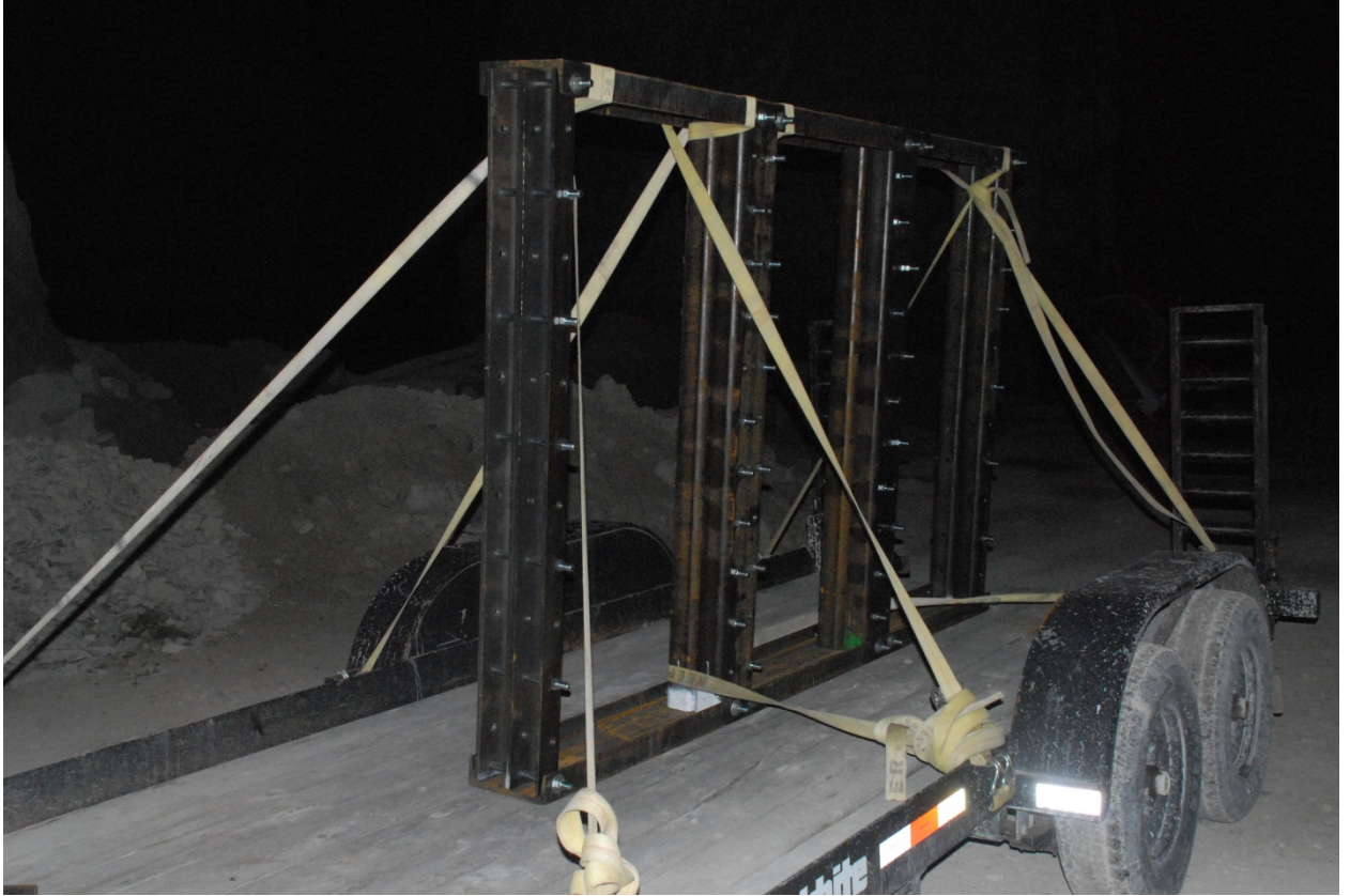
Figure 3.4. Steel Framing Assembled Off-Site
