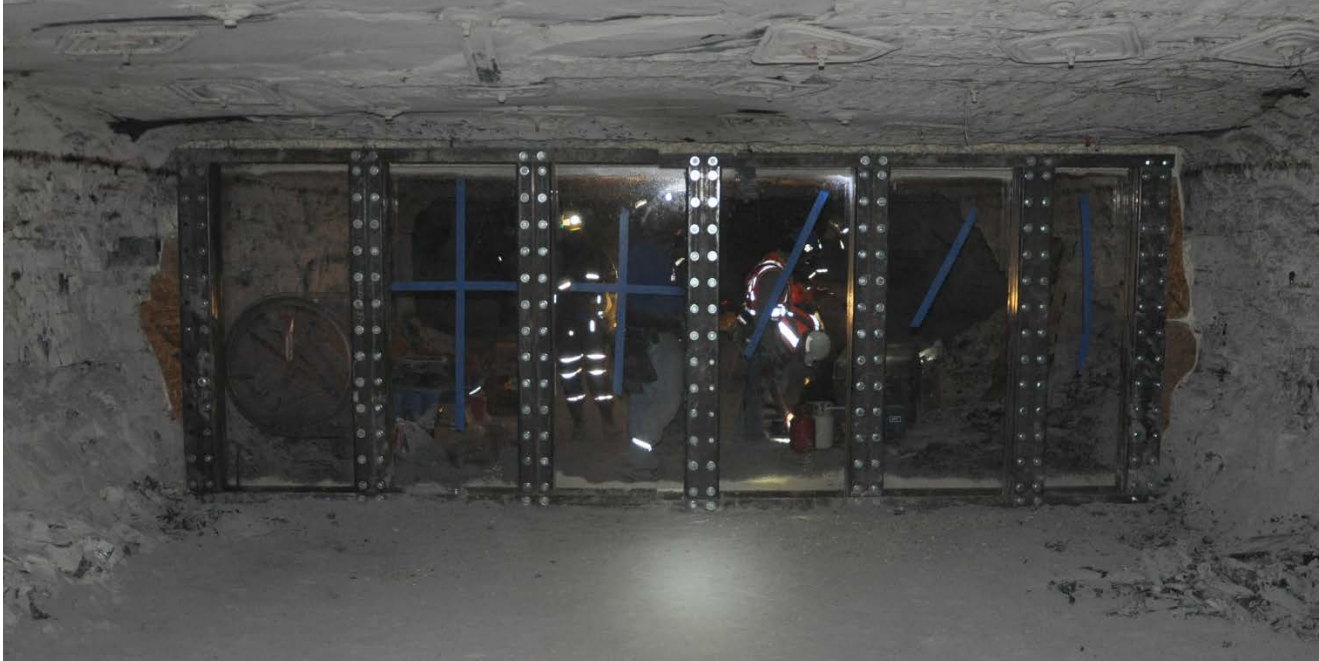
Figure 4.13. Final Sealed Installation Inside
