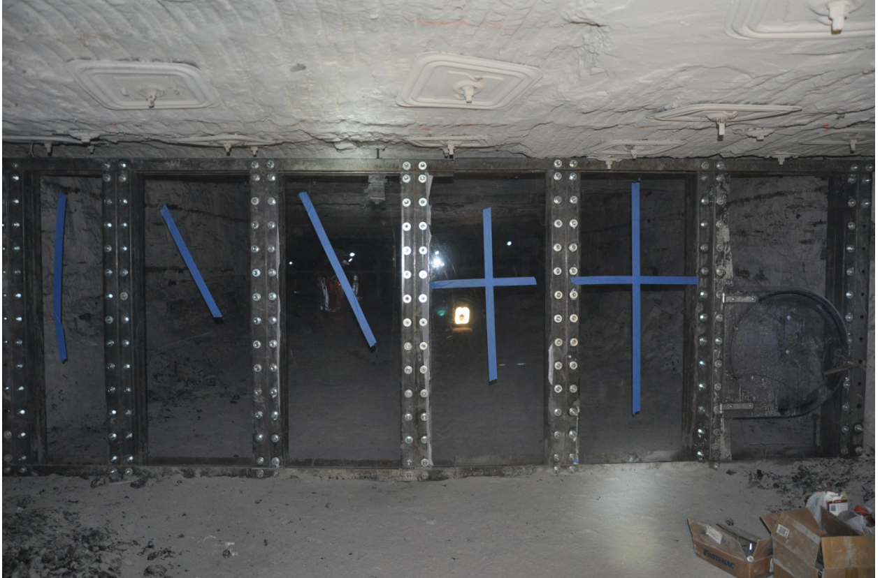
Figure 4.7. All Polycarbonate Panels Installed
