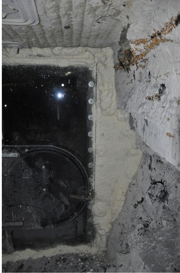
Figure 4.8. Mine Foam Covered Plywood Used to Seal the Wall
