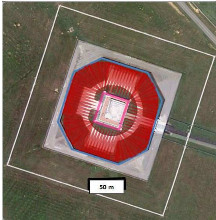
FIGURE 5.15: Aerial view of Fort Knox with possible deployment of sensor modules
