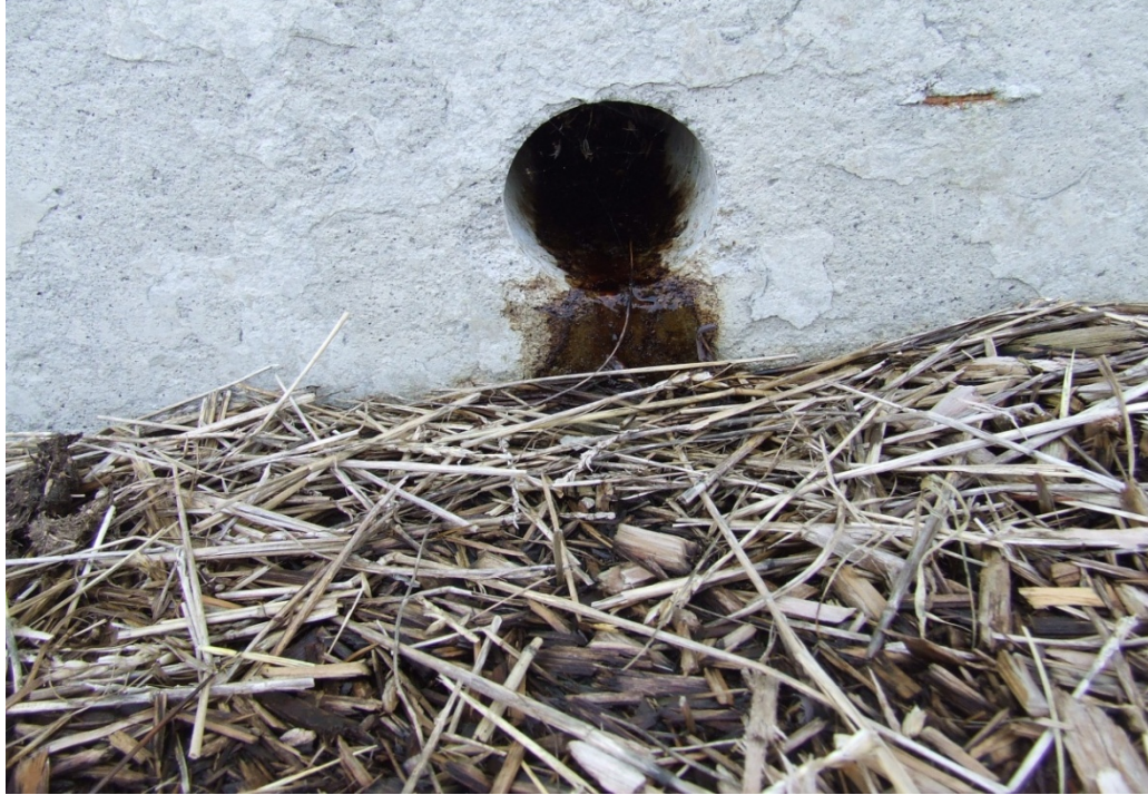
Figure 2.5: Hole in wall of X1, showing drainage from inside of pad.
