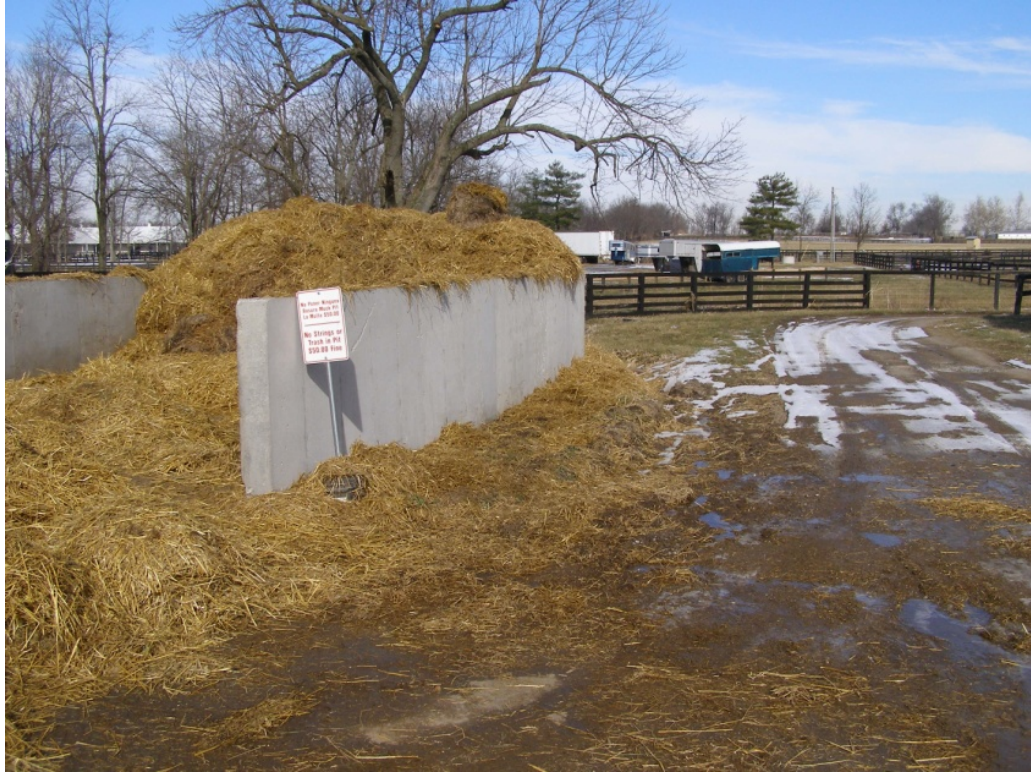
Figure 4.5: Spillage, mud, and tire dredging surrounding pad C2.
