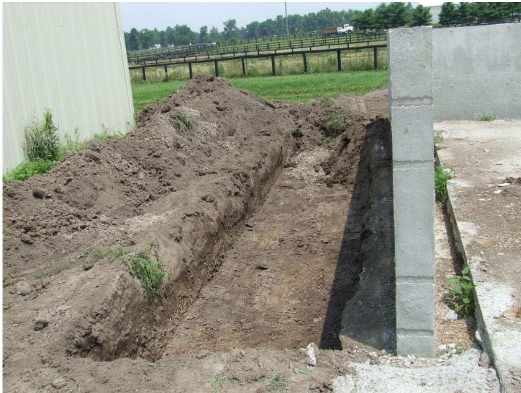
Figure 2.6: Excavation of rain garden basin at X1.
