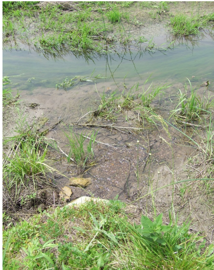
Figure 3.3: Groundwater seep in stream bank at Victory Haven.
