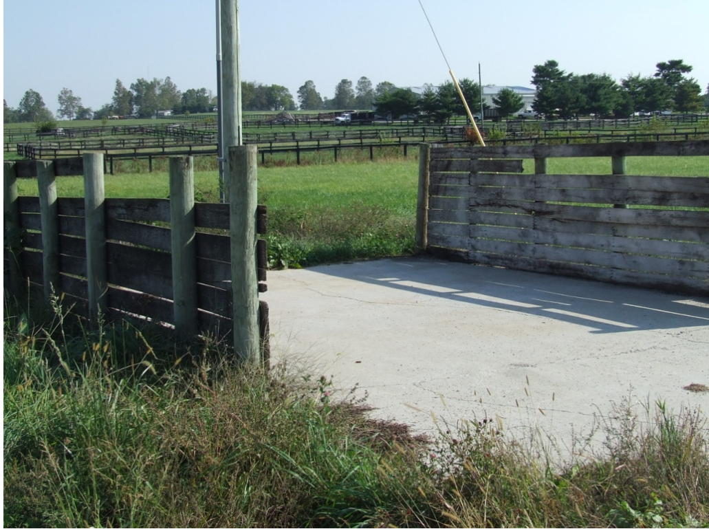
Figure 4.1: Old wooden-walled muck pad at Victory Haven.
