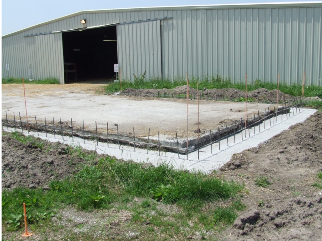
Figure 2.3: Beginning construction of concrete walls surrounding existing muck pad X1.
