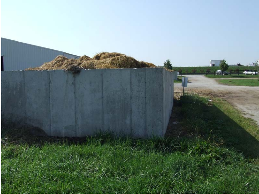
Figure 2.9: Control pad C1.
