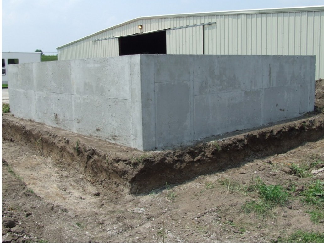
Figure 2.7: Excavation of rain garden basin at X1.
