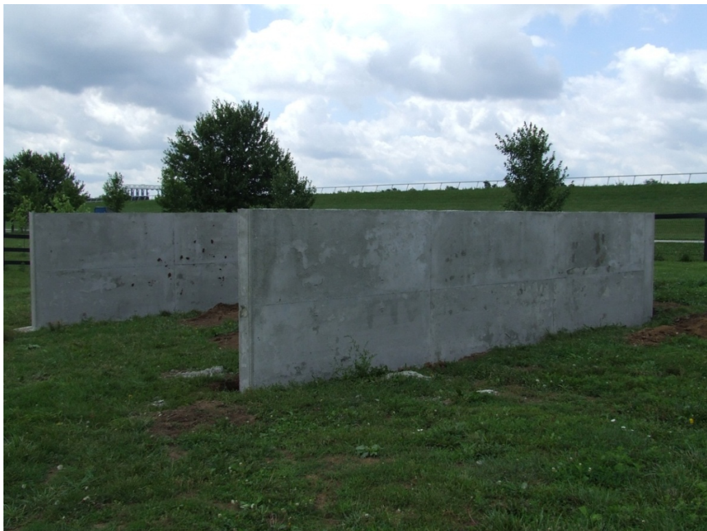
Figure 2.4: Completed walls at X2, before installation of new concrete pad.
