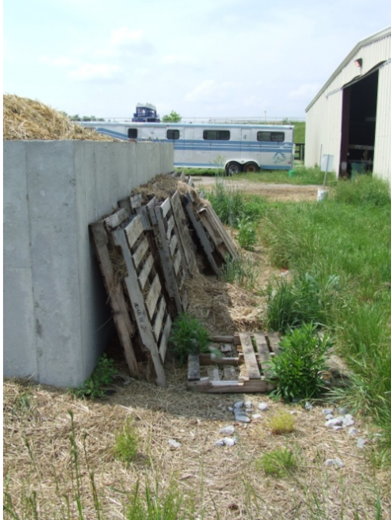
Figure 4.8: Overflow and wooden pallets stacked in the rain garden basin at pad X1.
