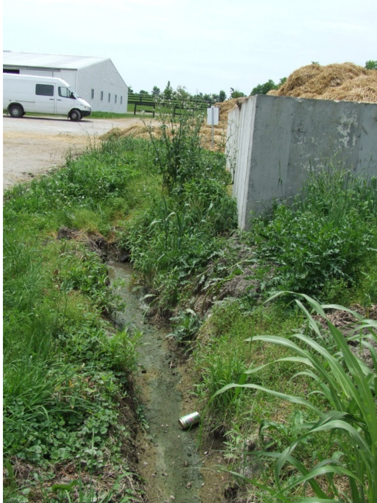
Figure 4.3: Drainage ditch leading runoff from C2 to nearby Cane Run tributary.
