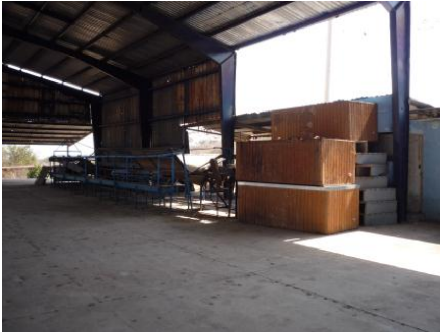
Figure 10-7 Inside of the abandoned packing facility Containers (“bathtubs”) were reminiscent of the uncompleted construction of HWT equipment. (Photo by author)
