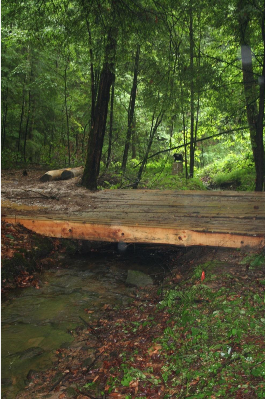
A.10. Bridge during storm event
