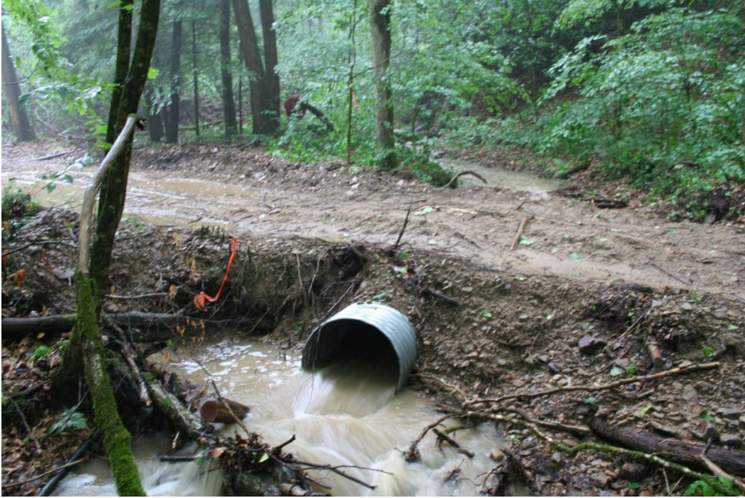
A.8. Culvert during storm event
