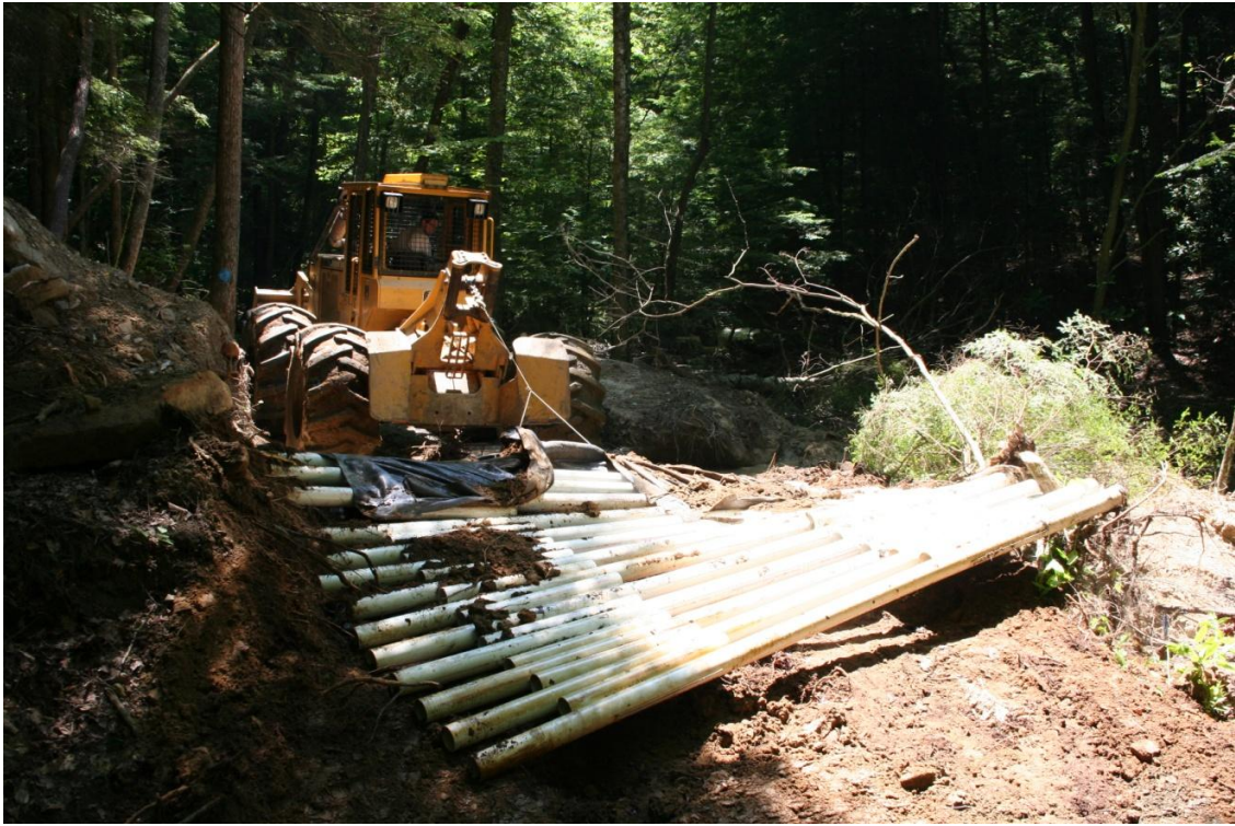
A.7. Pipe bundle after removal
