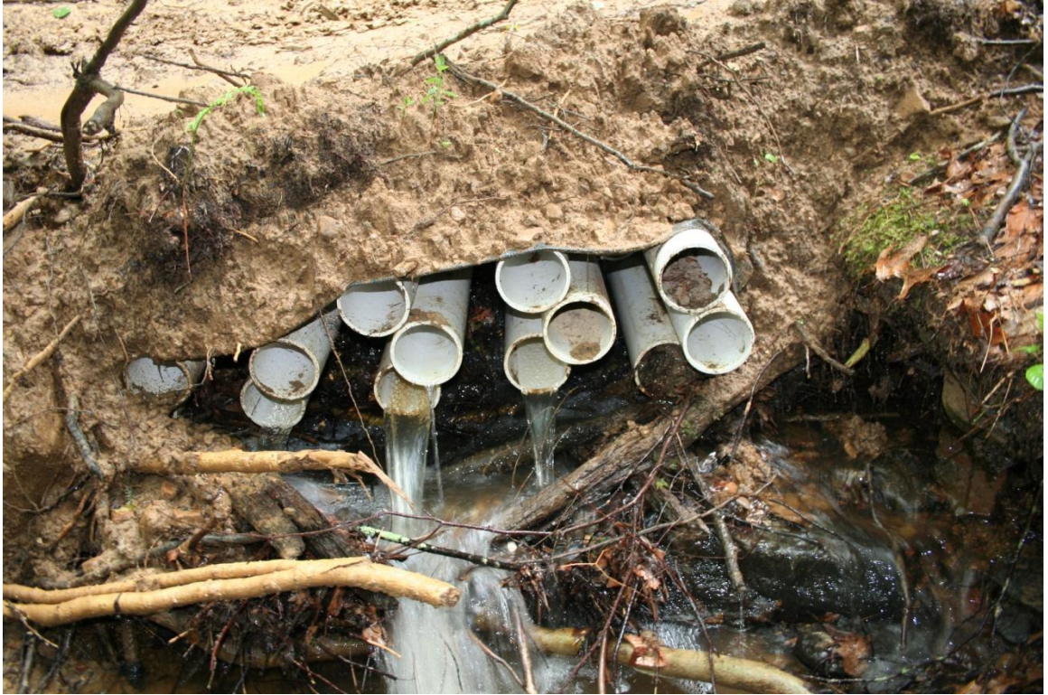
A.9. Pipe bundle during storm event
