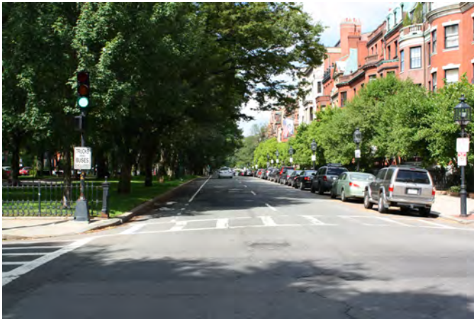
Figure 2.4: Commonwealth Ave. Bike Lane
