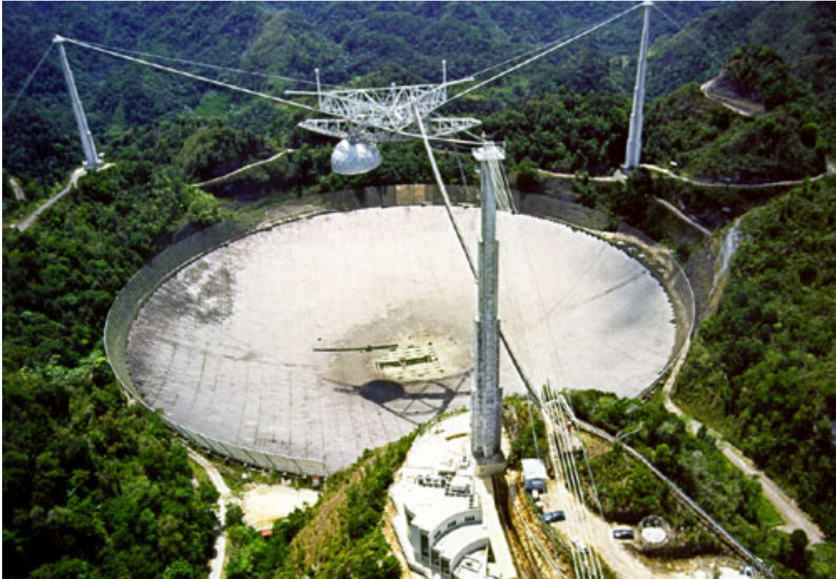
Figure 1.5: The 305-m Arecibo radio telescope, the largest single-dish radio telescope in the world, is located in Puerto Rico. Image courtesy of the NAIC - Arecibo Observatory, a facility of the NSF.
