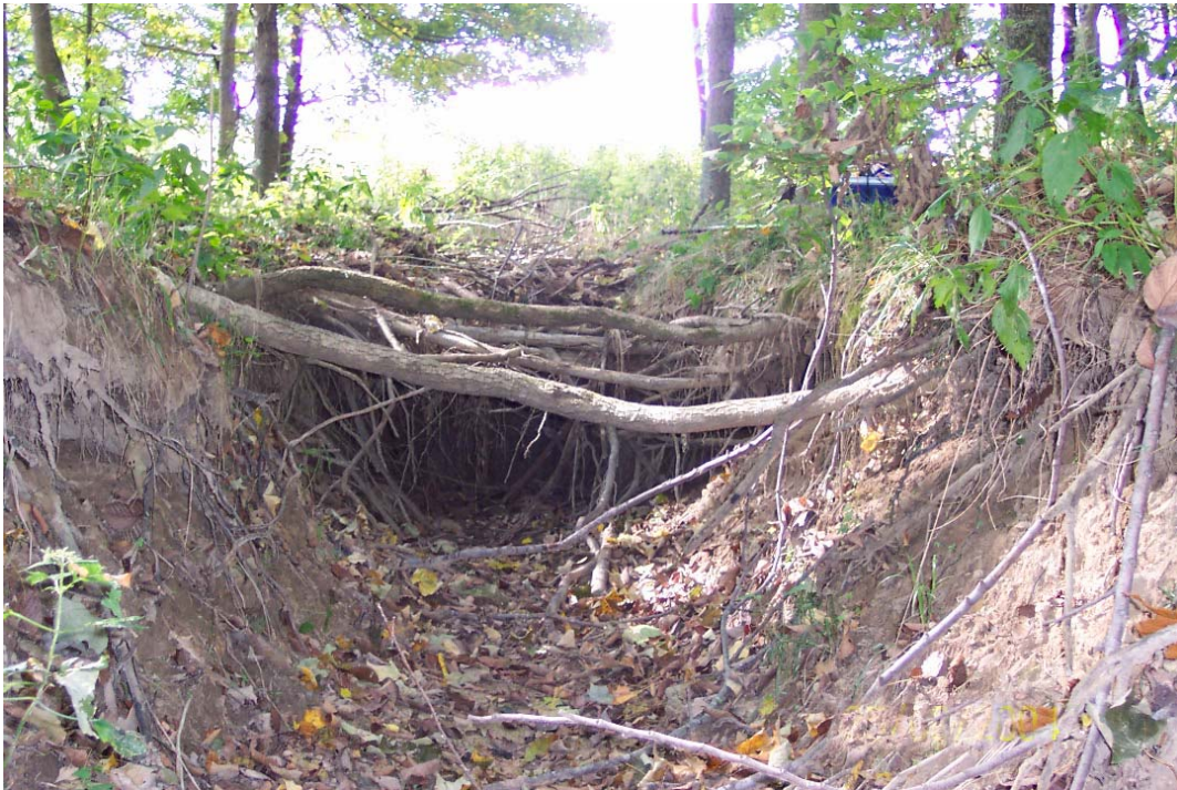
Figure 2.11. Roots create an overhang above a moderate-sized gully at the forest/grass boundary at the bottom of the main study area area. A blue and white cooler is visible through the brush. Photo by author, October 7, 2004.
