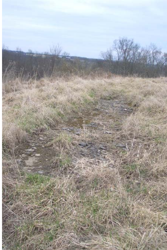
Figure 5.48. Exposure of bedrock along the grassed shoulder of the main study area. Photo by author, March 15, 2005.
