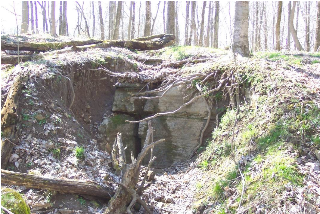
Figure 5.15. Relict shaft below Hillslope A, with widened vertical fracture through a Tyrone exposure in the uphill wall. The shallow eroded channel above the fracture passes over and within a 40-50 cm deep layer of bentonite. Current sediment movement processes are removing the soil lying to the left of the rock wall in the photo. This soil bank fills in the gap between the exposed rock wall shown here and a second exposed wall lying outside the photo range. Five such walls and intervening soil banks surround a central open area at this site. Photo by author, April 2005.
